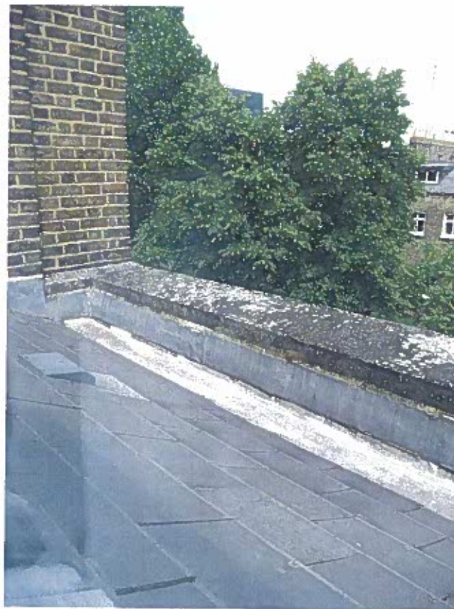
Photo 10: Taviton Annex (No. 11 Taviton Street) Rear Coping.
