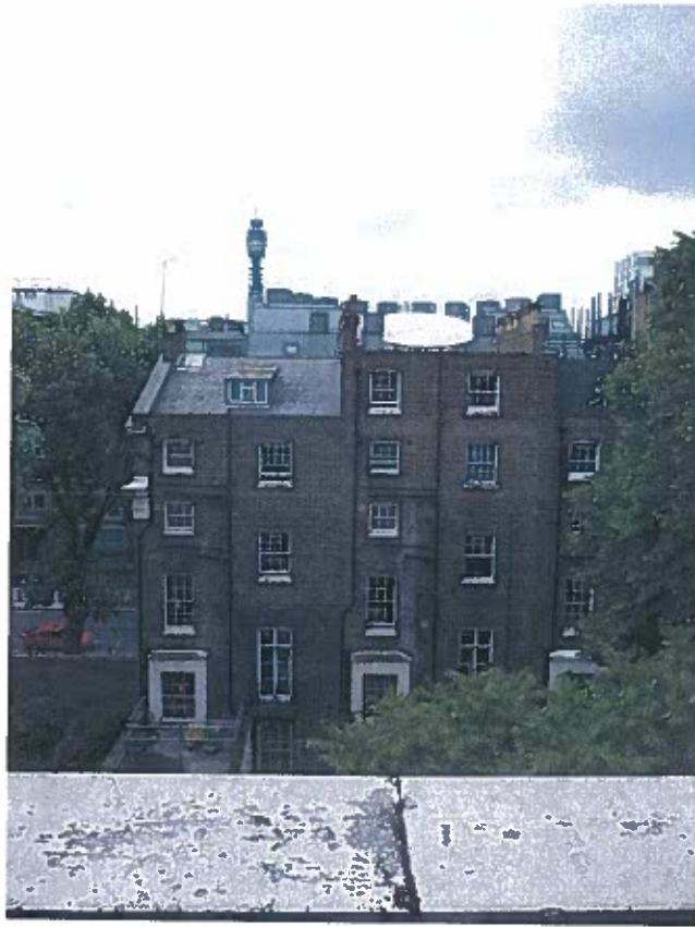
Photo 9: Taviton Annex: Rear Elevation
