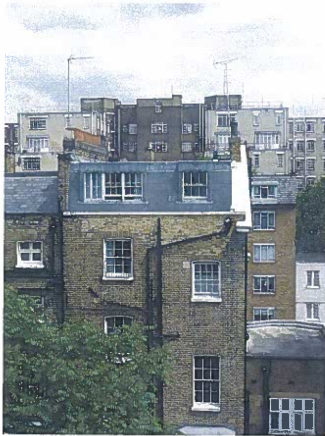
Photo 11: Endsleigh Annex: Rear Elevation
