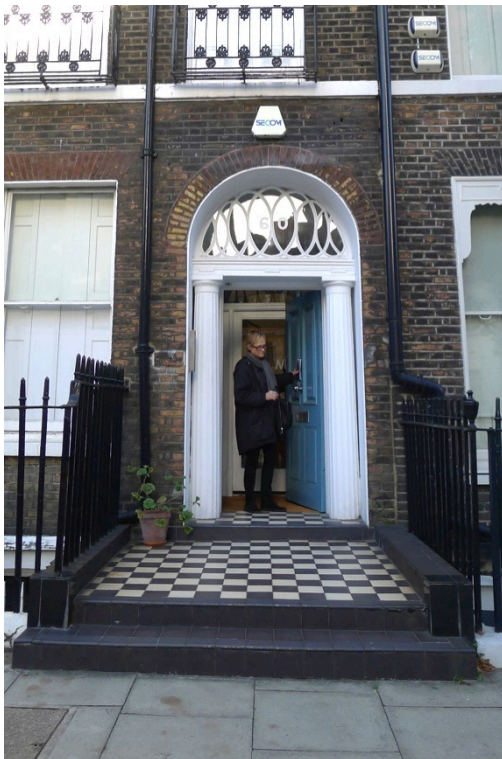
3. n.60 Doughty St. in 2013, before completion of the refurbishment works. Railings on the right kerb were already missing
