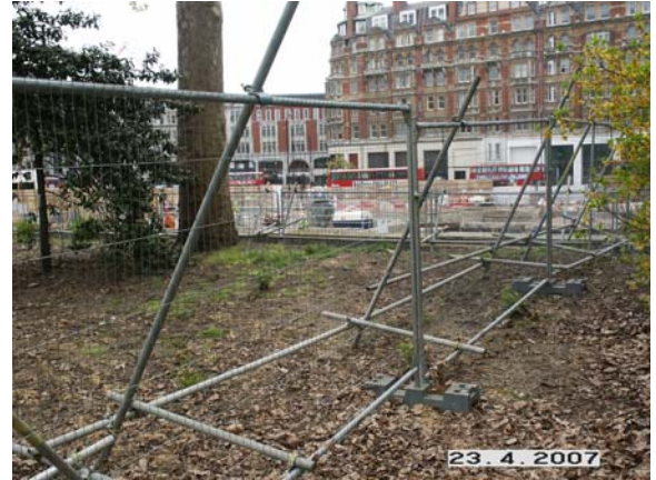
Effective fencing in position
