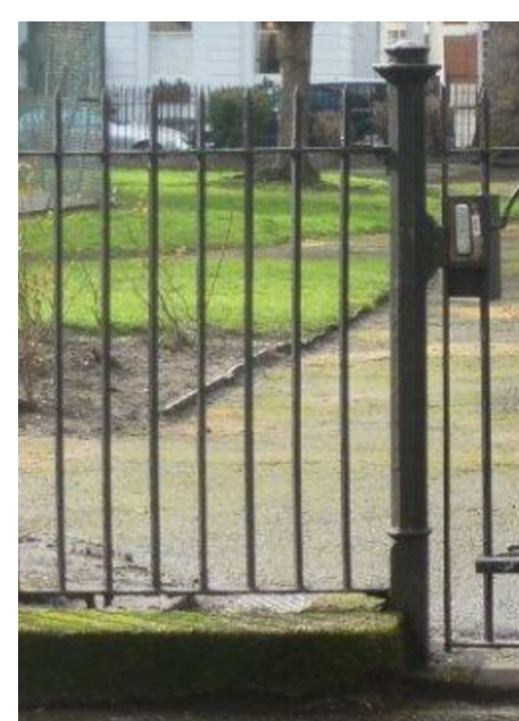
Existing Garden updated, railings & pointed finial
