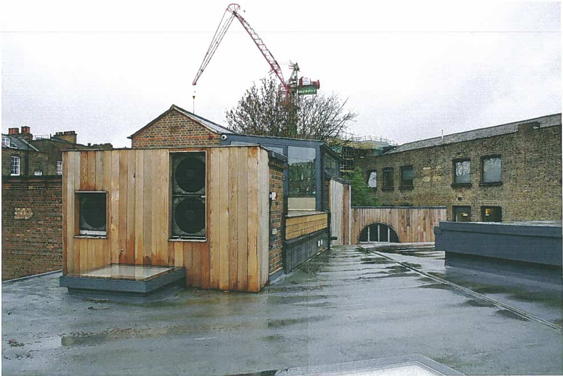
1 - VIEW OF EXISTING TIMBER SCREEN & VISIBLE ASHP FANS ON ROOF
