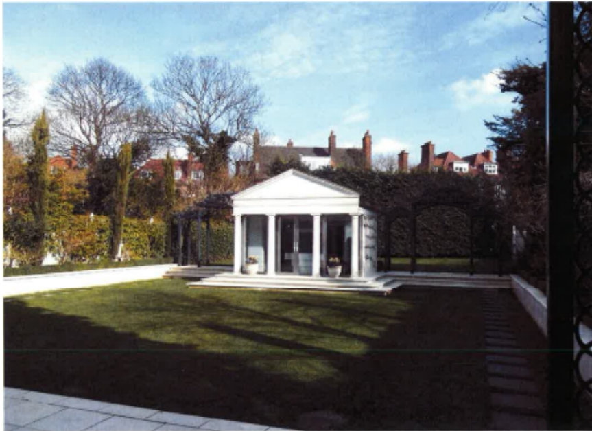
Rear garden showing the existing summer house
