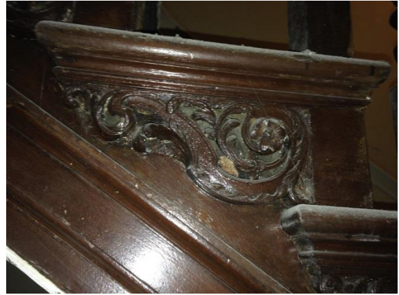
Typical Bracket Detail – Ground to Second Floor
