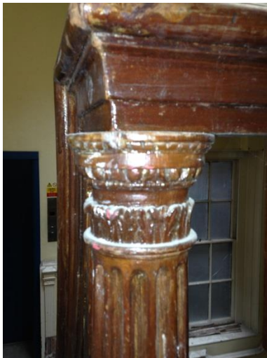
Detail to top of Newel Posts
