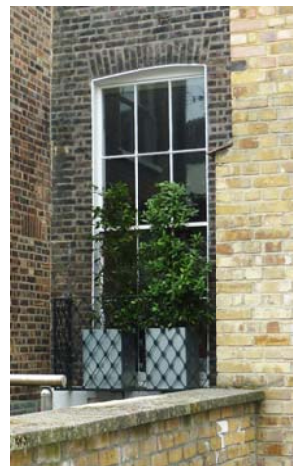
③ CAST IRON JULIET BALCONY (SAME NEXT DOOR, vertical railings instead of diamonds pattern)
