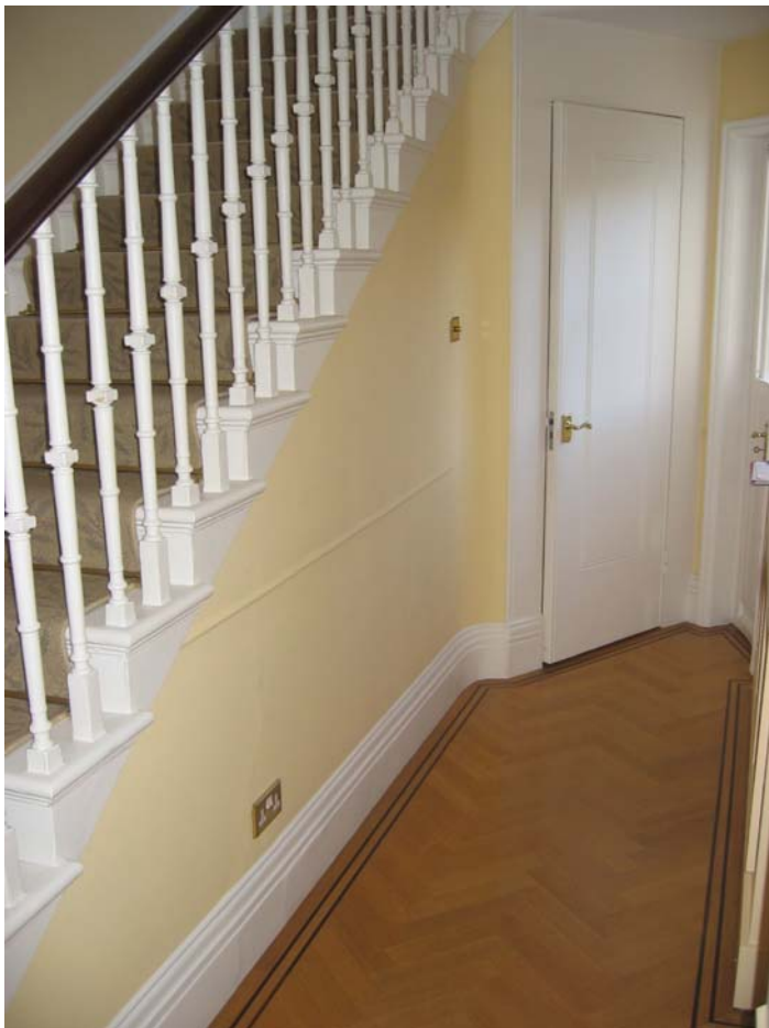
Main stair at raised ground floor
