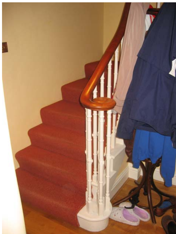
Overclad stair at No. 21
