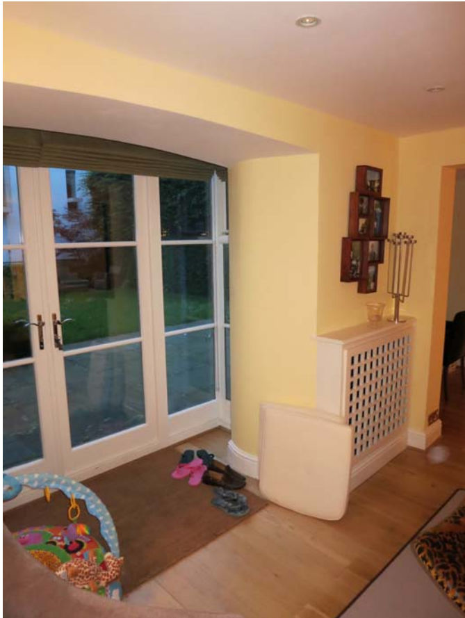
Opening widened, downstand beam & ceiling to be raised
