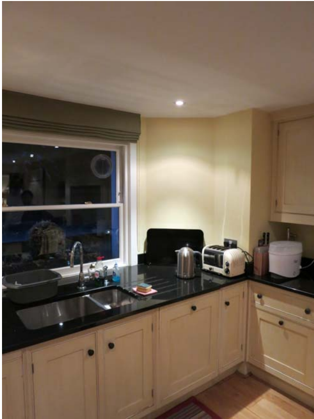
Masonry panel where window proposed to be added.
