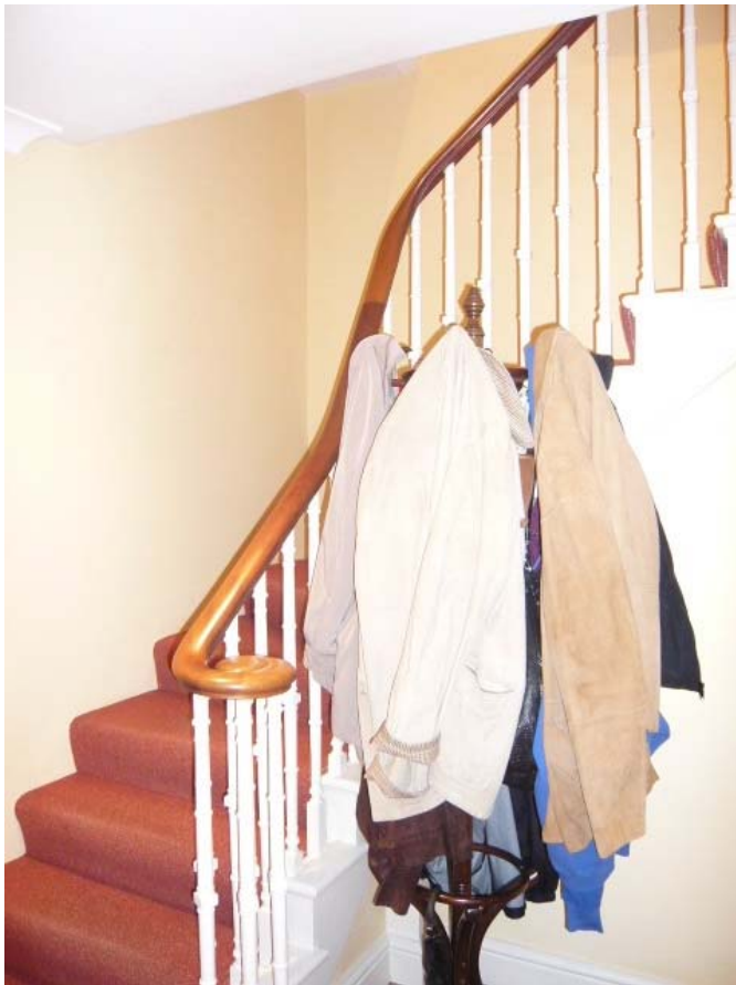
Basement stair from bottom, (inadequate head height over)
