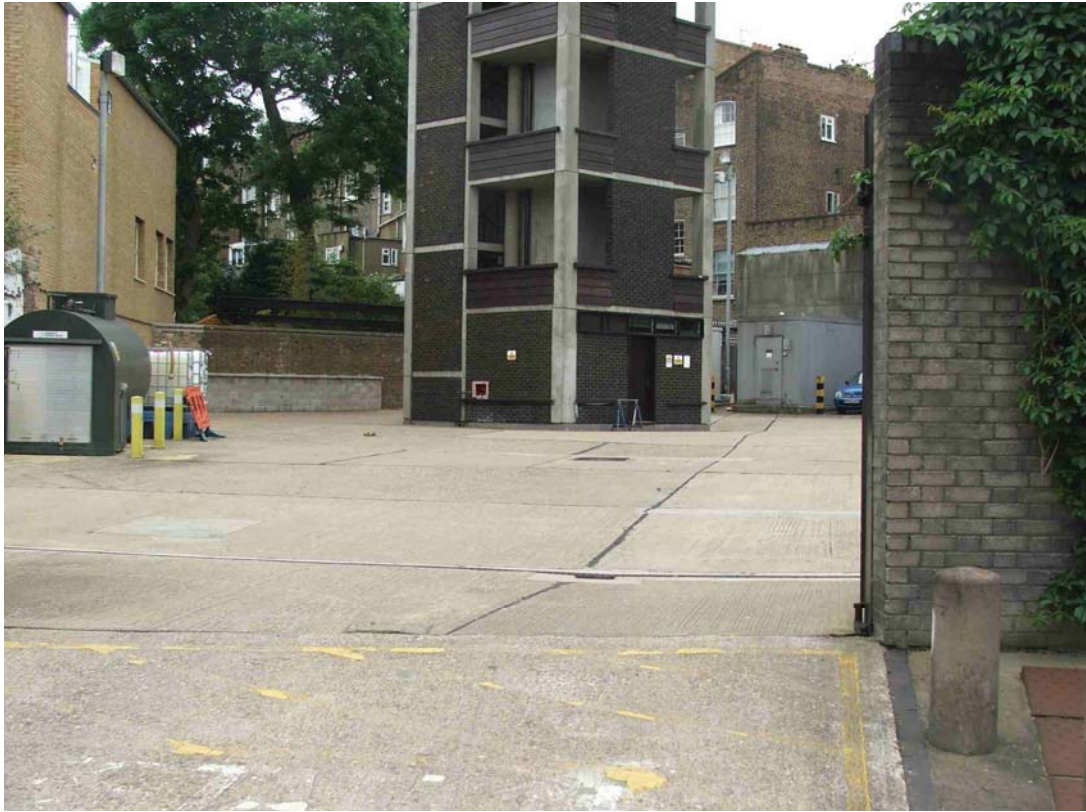
Figure 3.7: Off-site Fire Station, with fuel tank (LHS), practice tower (C) and generator (RHS)
