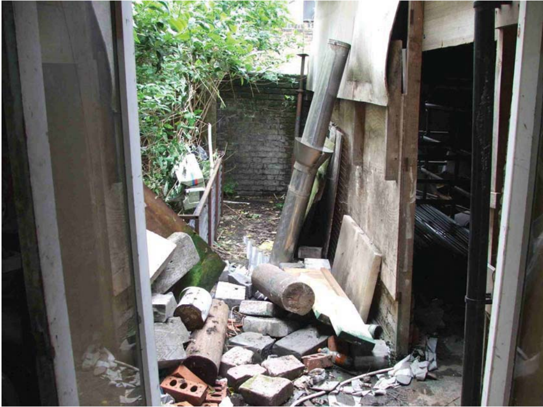
Figure 3.3: View of yard area with lightwell to left, outbuilding to right
