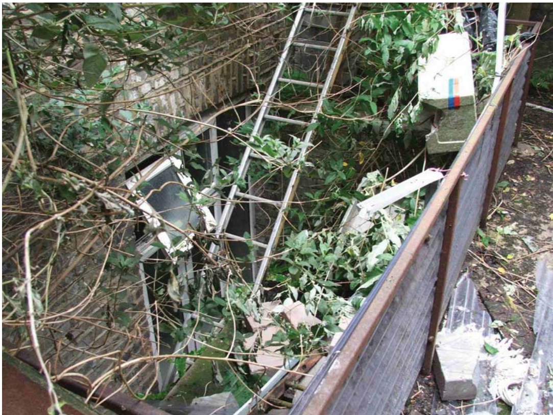
Figure 3.4: Lightwell to basement area (in yard)
