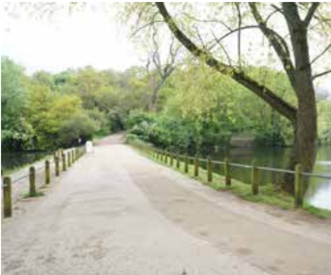
Existing view looking north east across the Mixed Bathing Pond dam crest. The proposed works will raise the dam by 0.5m with a further 0.5m grassed bund along the upstream edge of the footpath.
