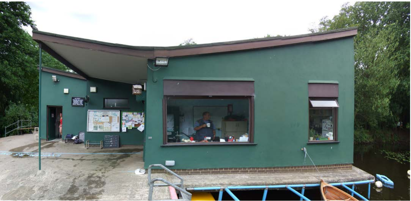
Figure 3.7 Limited window area obstructs lifeguards' sight line of the pond. Bulky roof profile
