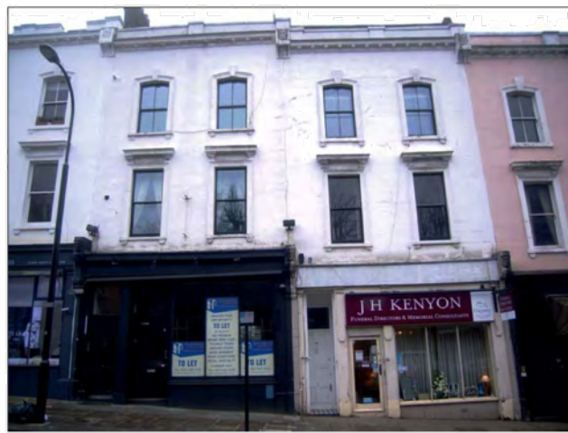
7 (left) and 9 (right) Pond Street – South (front) Elevation
