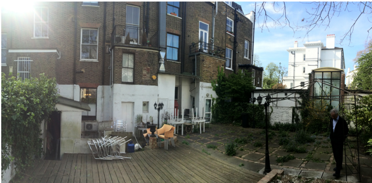
7 (right) and 9 (left) Pond Street – North (rear) Elevation showing the unification of the two properties and permitted changes to the rear fenestration etc
