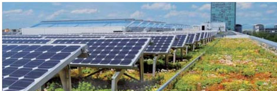
Green roof with PV panels
