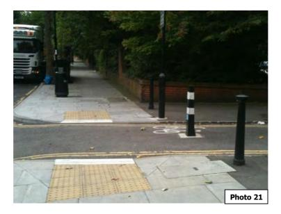
1.43 Barker Drive is a lightly trafficked residential road with cul-de-sacs and therefore provides a safe environment for pedestrians. **Photo 22** shows the presence of recently installed tactile paving and dropped kerbs which are in good condition and of a shallow gradient to assist mobility impaired users. There is also regularly placed street lighting and natural surveillance created by the surrounding residential properties.
