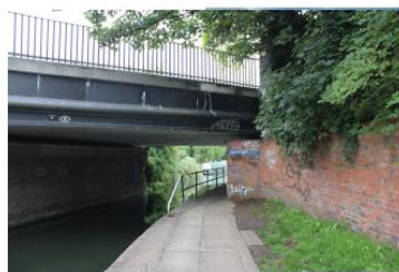
View of existing canal tow path
