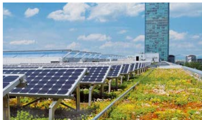
Green roof with PV panels
