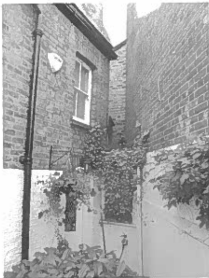
3 : The three storey brick structure that constrains the outlook from the rear of 3 Bisham Gardens
