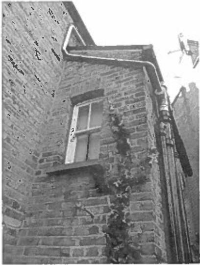
2 : a small rear extension accommodates a staircase
