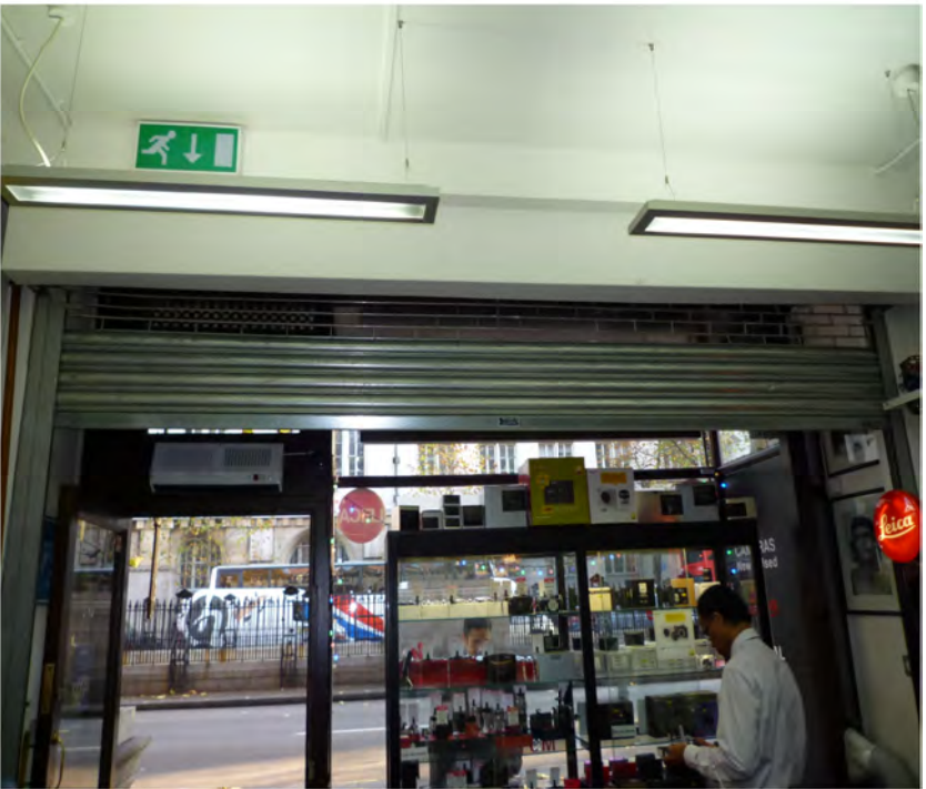
PHOTO 3 : The in situ internal roller security shutter "Brick Bond Pattern" as existing to the adjacent retail Unit 29 Southampton Row.
