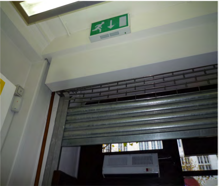
PHOTO 4 : The in situ internal roller security shutter showing the fixing points to the wall and not on the ceiling therefore avoiding the existing listed features.
