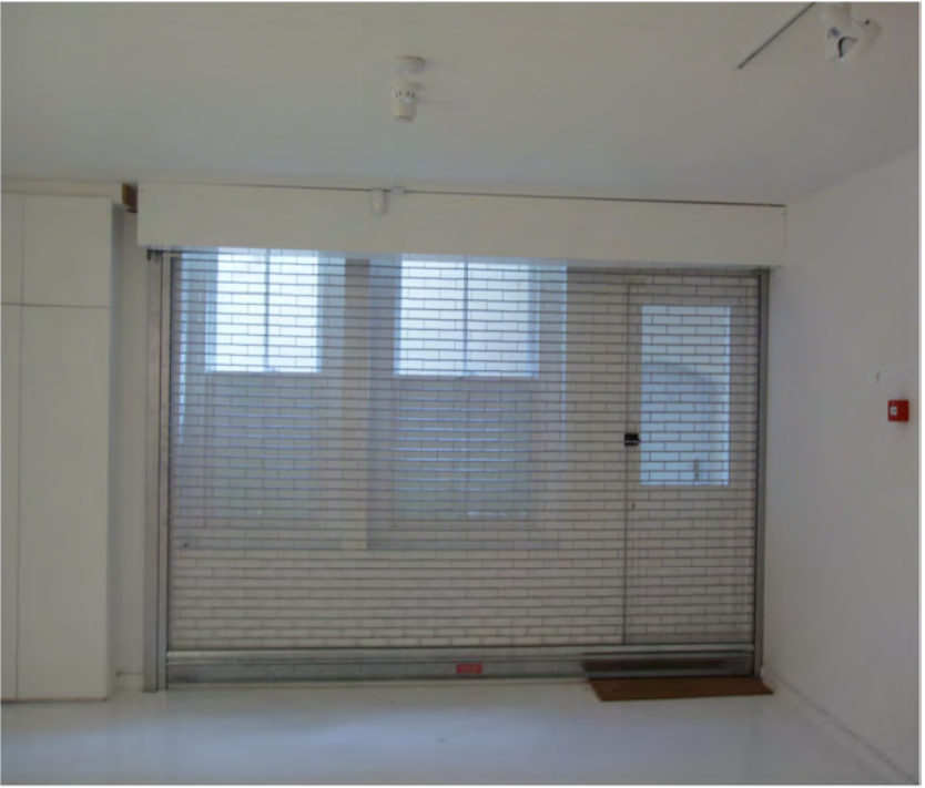
PHOTO 1 : Example of the internal roller security shutter installed "Brick Bond Pattern", internal view.
