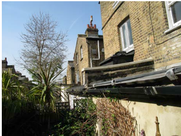
LOW REAR BUILDING TO BE REBUILT
