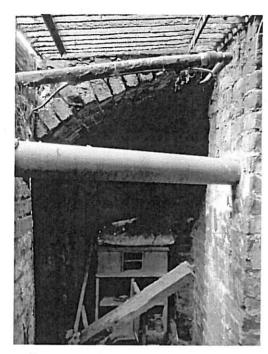
13 Existing External Lightwell: Currently the external lightwell is obstructed by service pipes and is in a poor state of repair.
