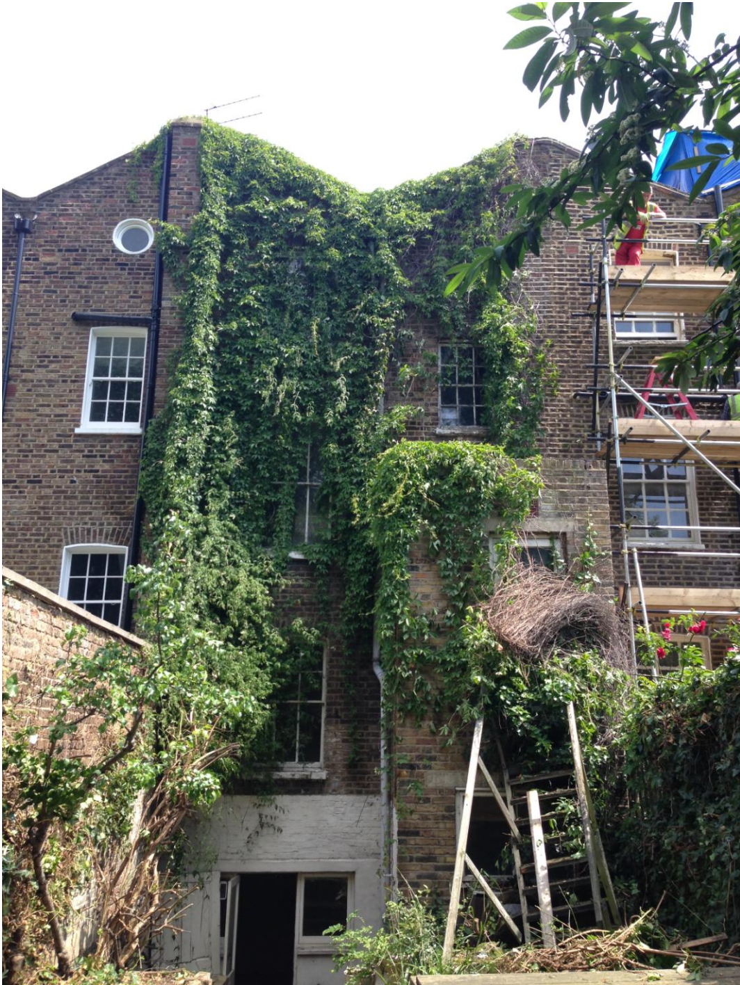
Photo showing existing rear elevation
