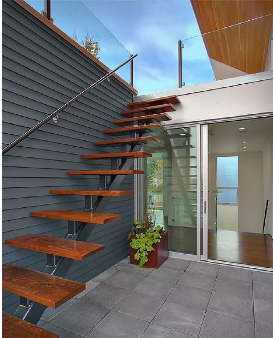
Image showing a similar staircase as proposed with a central steel core
