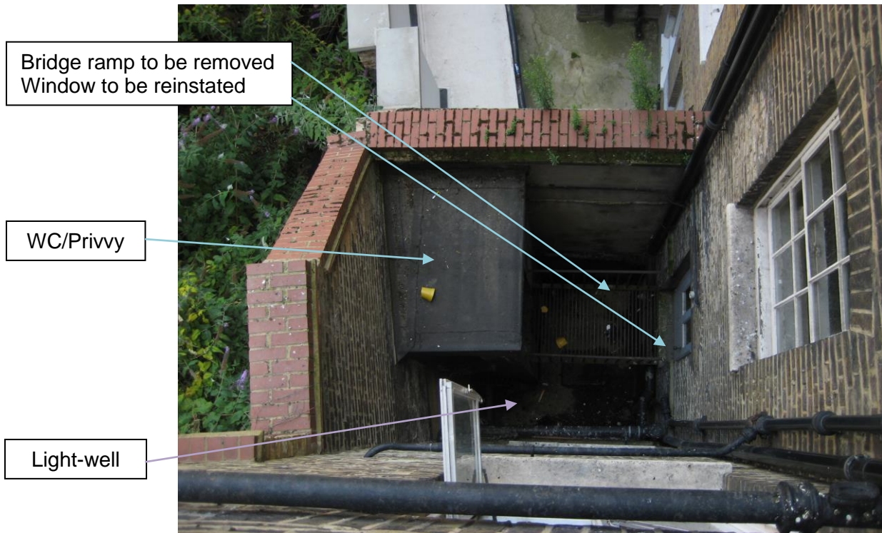
Fig7: Photo of WC/privvy block from above (LP Architects 2014)
