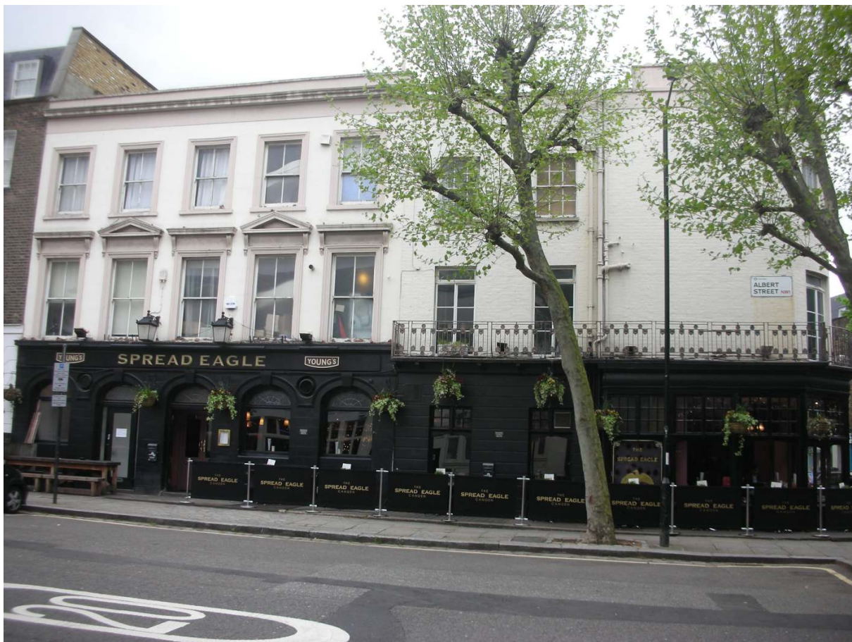
Photo A – East facing side elevation onto Albert Street.
