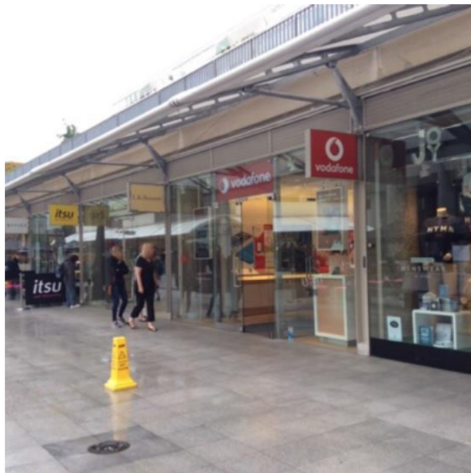
Front façade – Vodafone Unit 20 Brunswick Centre, London.
