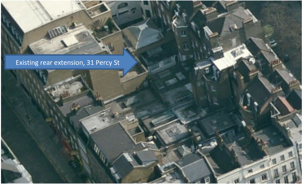
Figure 7. View of development to rear of Percy Street properties.
