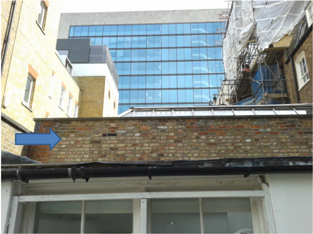
Figure 3. Boundary wall of adjoining rear extension to east
