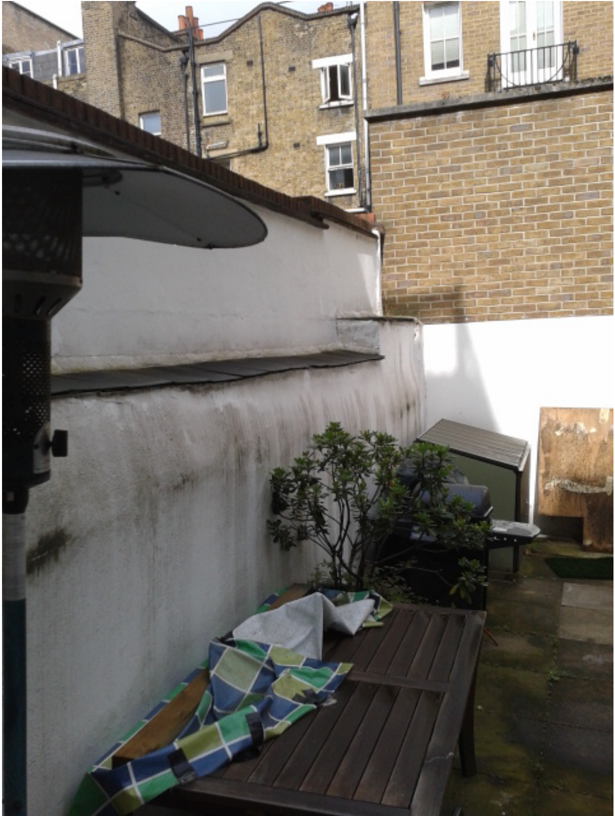
Figure 4. Adjoining boundary wall of extension to rear (right side of photo) and adjoining boundary wall of extension to west (left side of photo)
