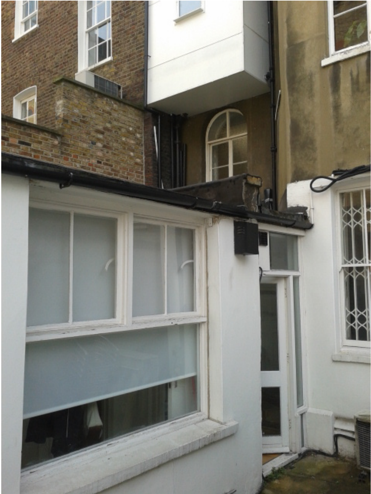
Figure 1. Existing single storey lower ground floor rear extension (bottom left) and rear elevation of original building (right).
