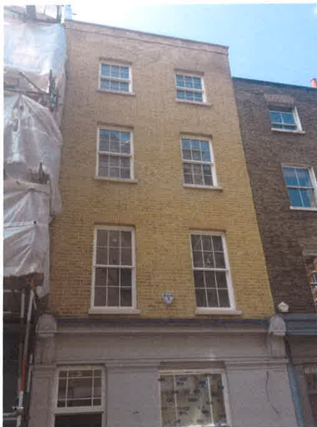
Photograph 1: Front elevation of 7 Coptic Street
