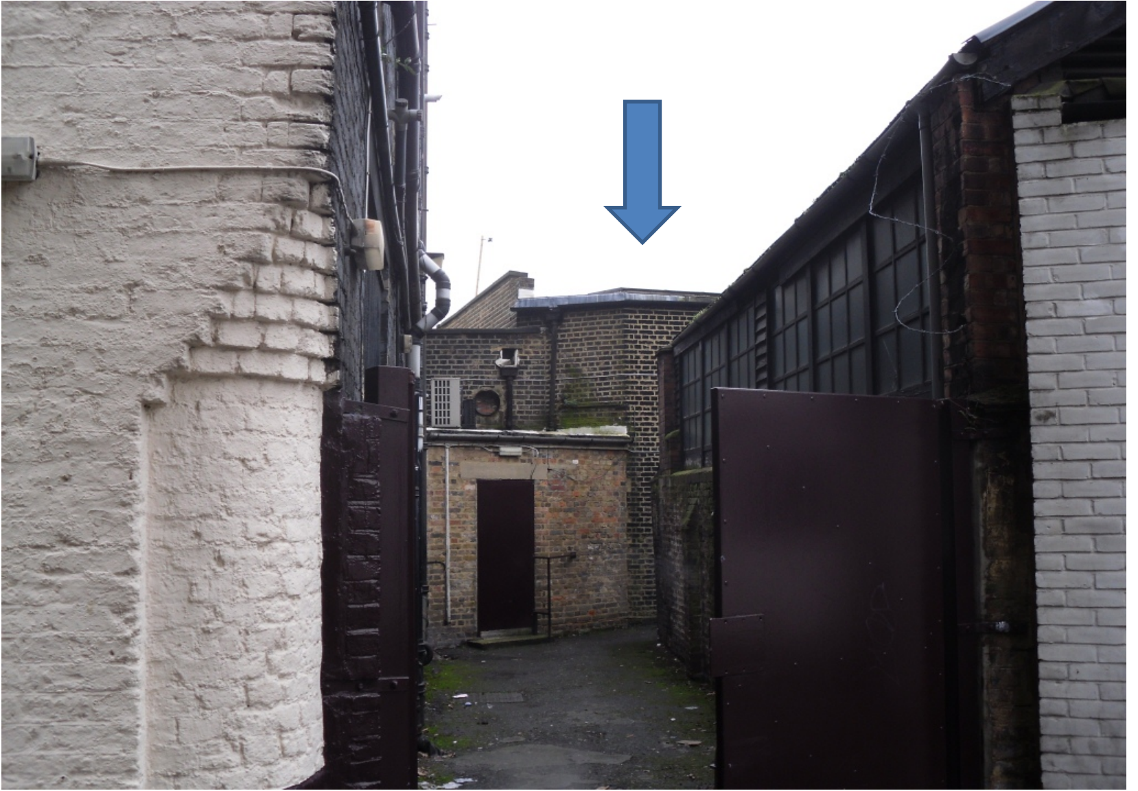
Rear of double height closet wing
