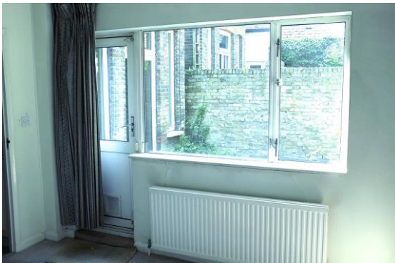
Interior view of the existing rear extension to be removed
