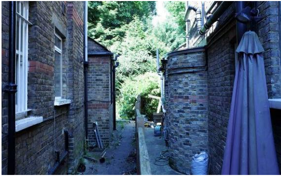
View looking down the side alley, as existing
