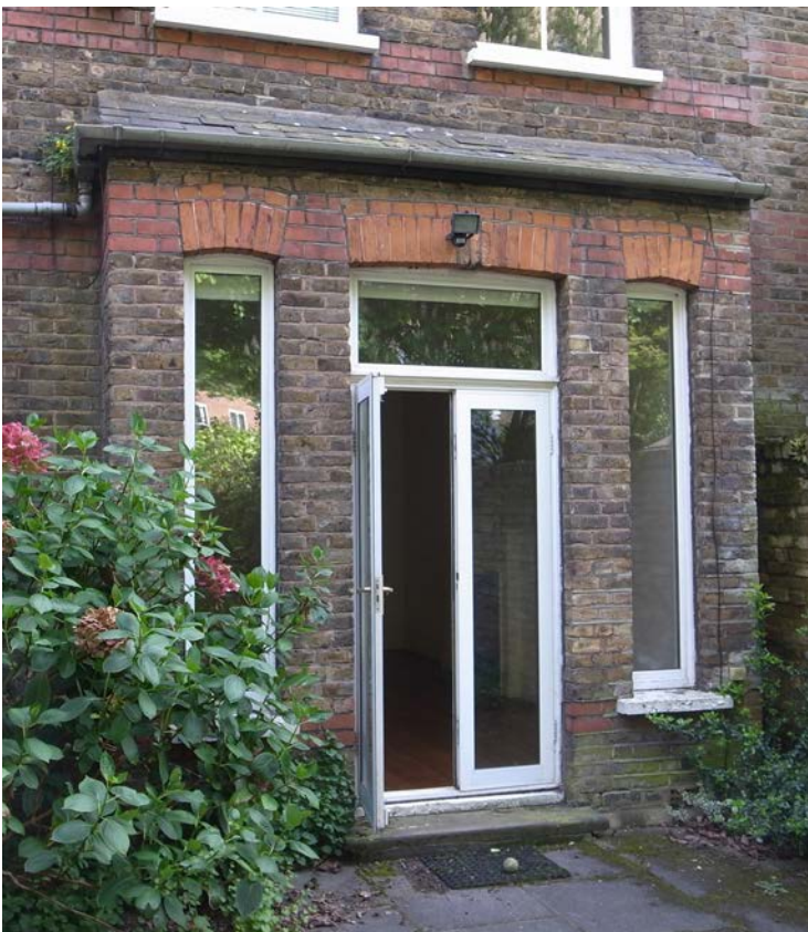
Bay window (to be demolished)
