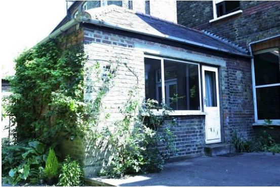
The existing rear extension, showing inserted window and door
