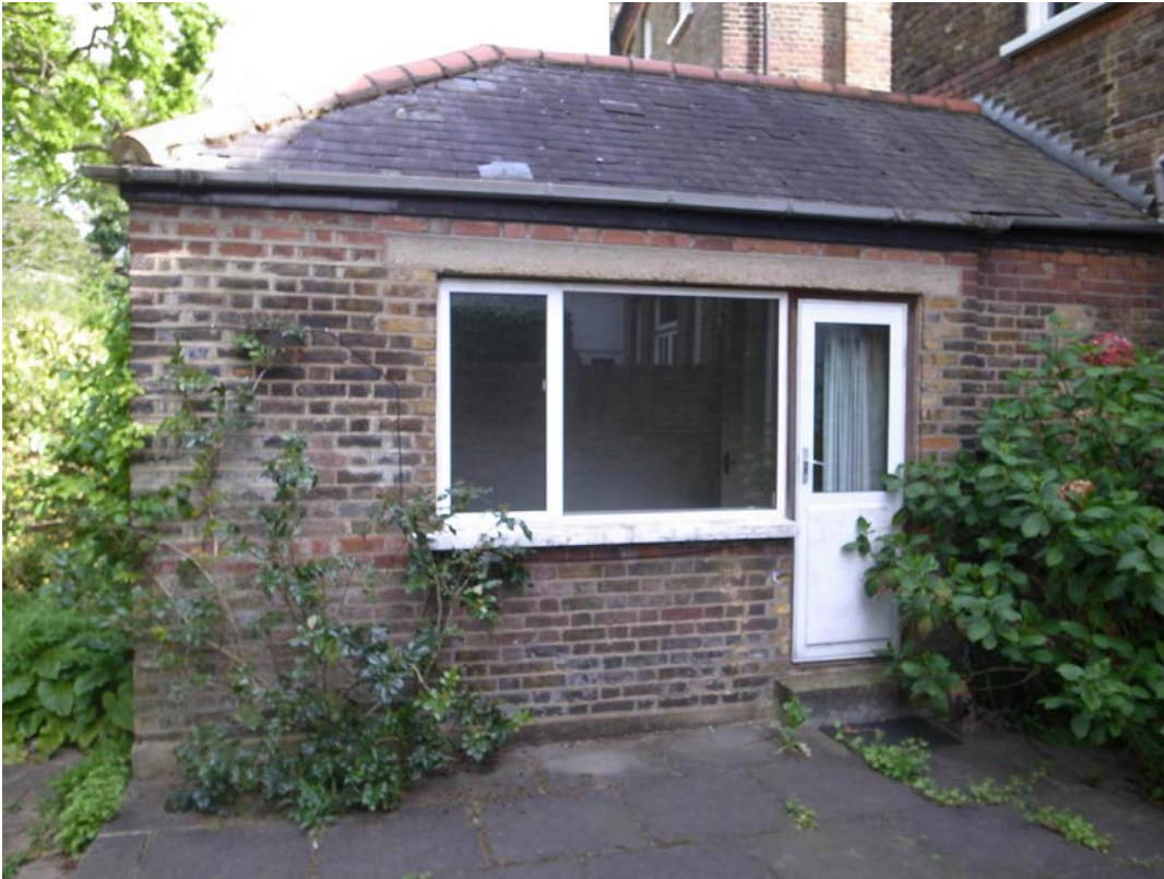
Rear addition (to be demolished)
