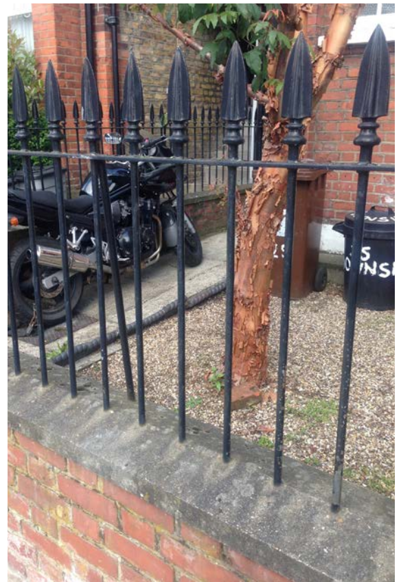
Railings to 25 Downside Crescent
