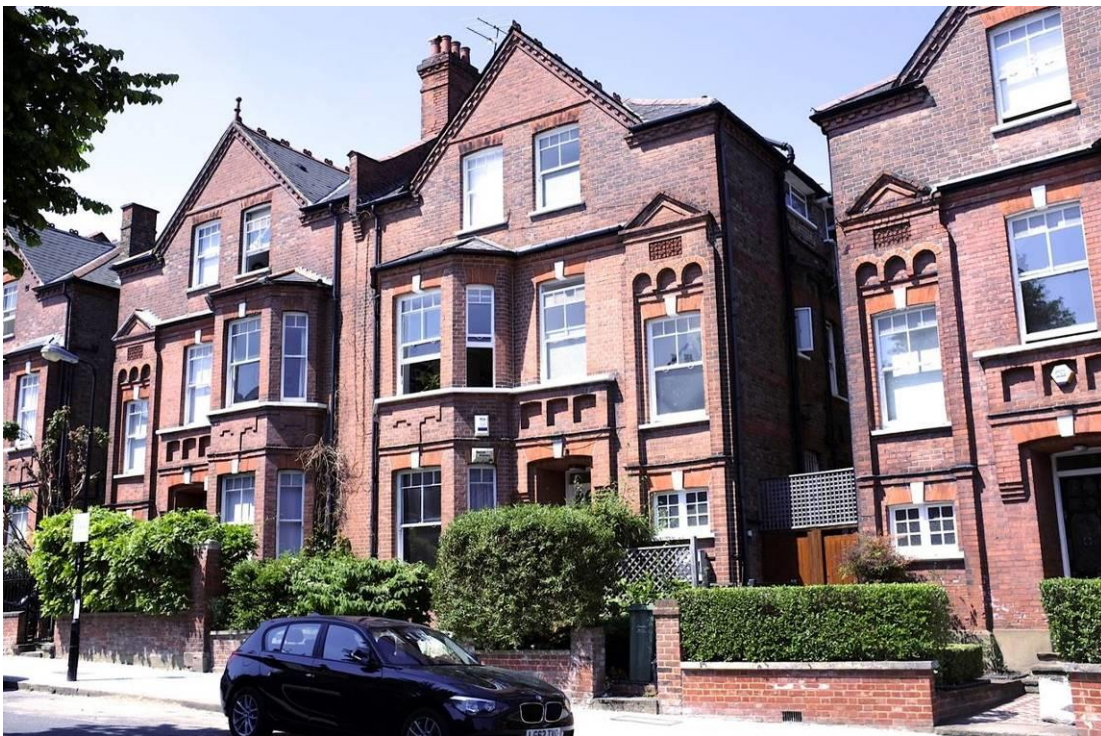
View of the application site, showing the gates and trellis in the typical narrow gap between the semi-detached pairs
