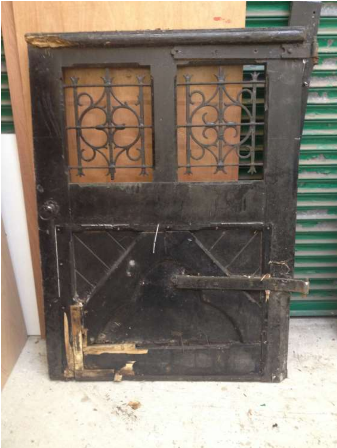
Rear of existing gate
