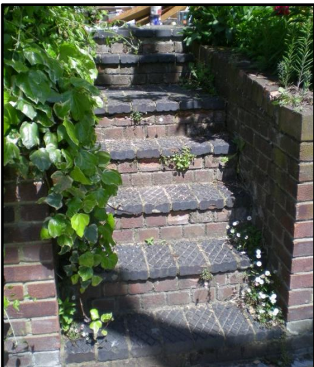
Fig 3: Existing stepped access
