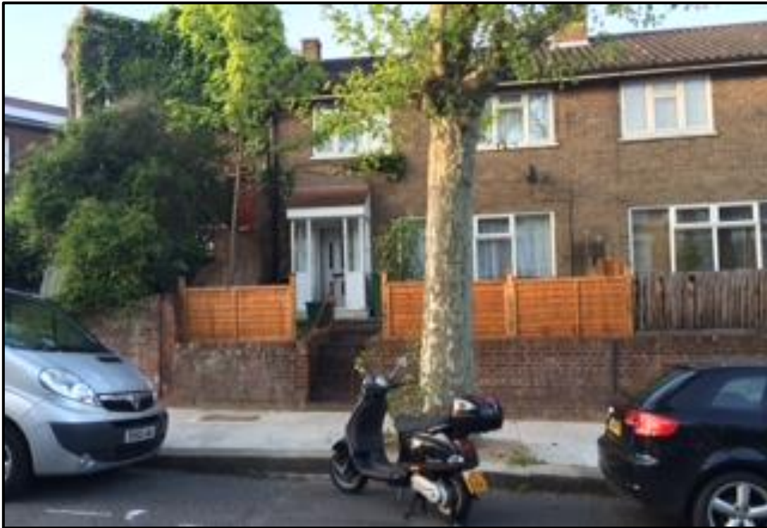
Fig. 2: Front elevation of 6 Westbere Road, NW2 3SR
