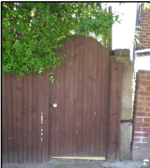
Fig. 5: Existing rear access gate
