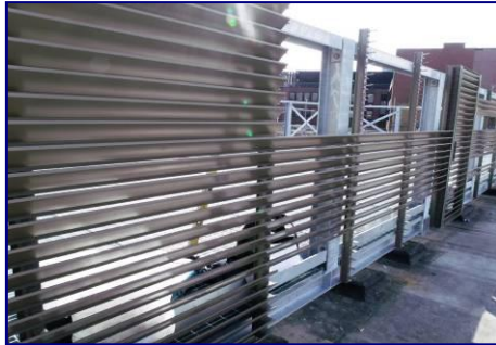
Figure 10: Part installed louvres.
