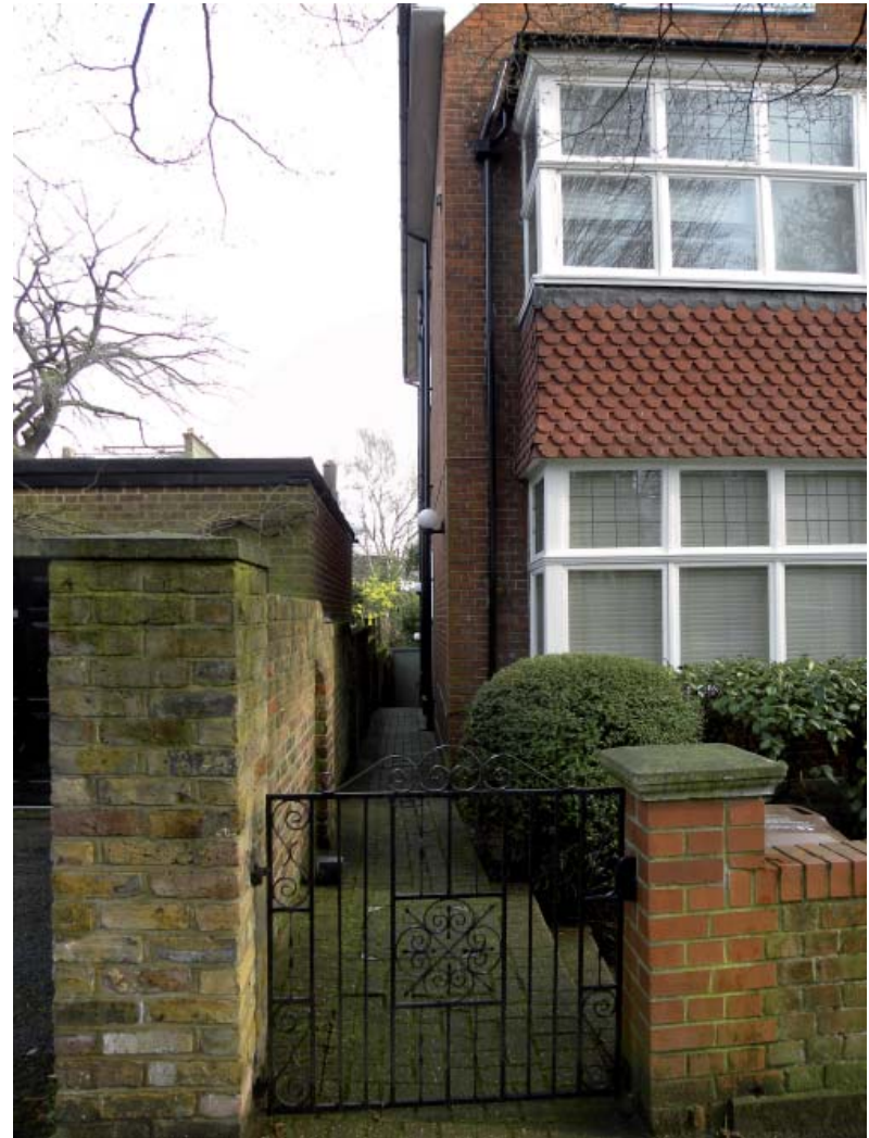
Side View of No 14 Eldon Grove
