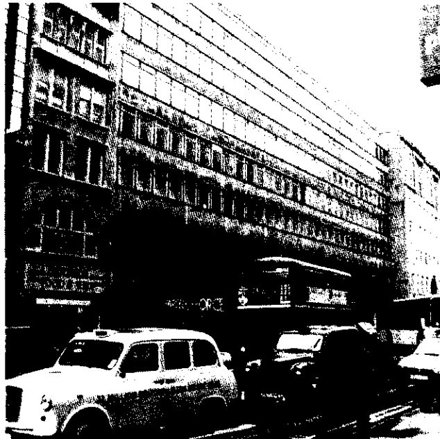
Continuous Vehicle Congestion On High Holborn. The Stone And Glass Facade Of Procter House Is Currently In A State Of Disrepair.
