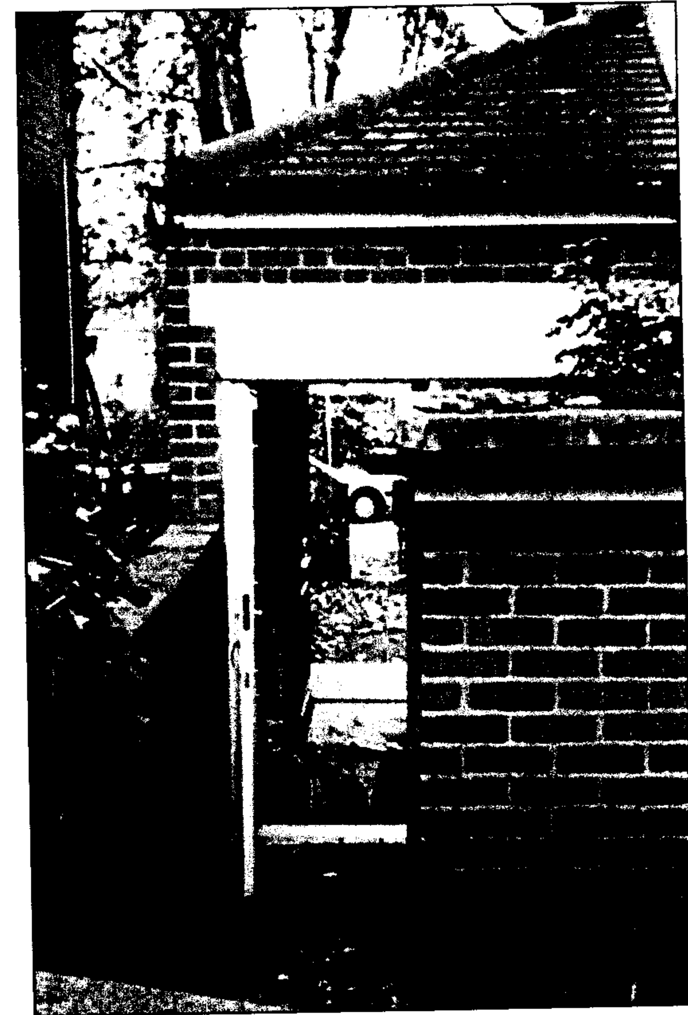
Above: view from the existing bin store in the side passage behind the entrance.
