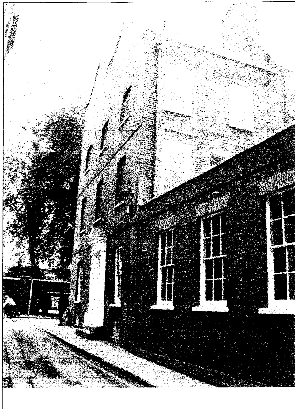
POSITION 1 VIEW FROM CENTRE OF ROAD KINGS MEWS
