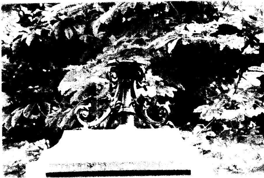
figure 2b. Missing 'Orb' to top of right hand pier at Swains Lane
