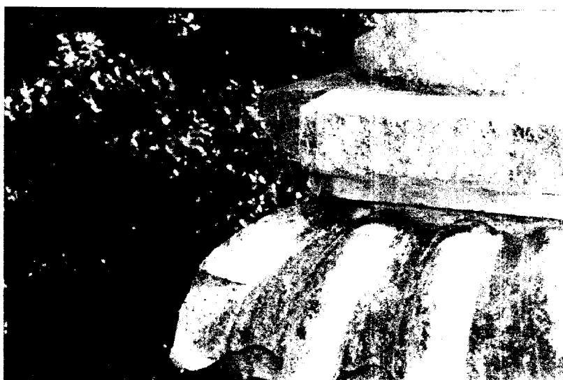
figure 11. Missing sections to Shepherd's base at top of Plinth
