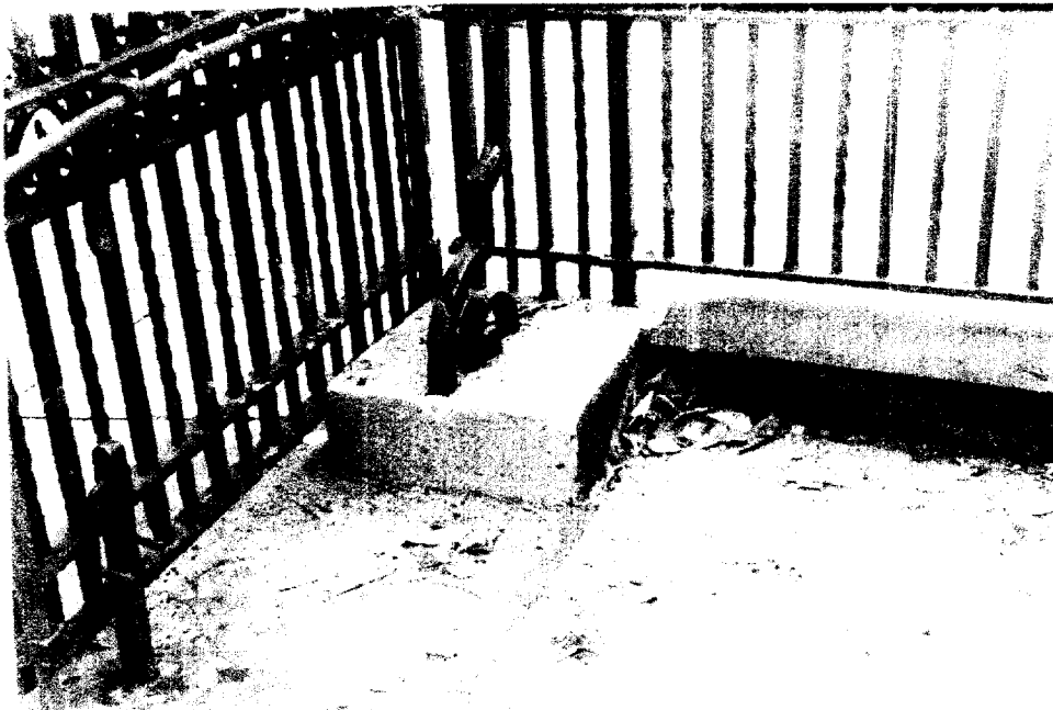
figure 5. Coiled backstay detail to left of Highgate Hill Entrance
