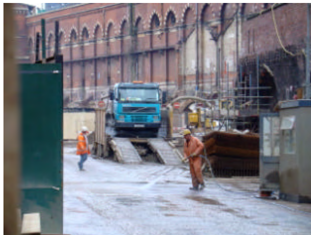
Figure 8: Illustration of wheel washing
