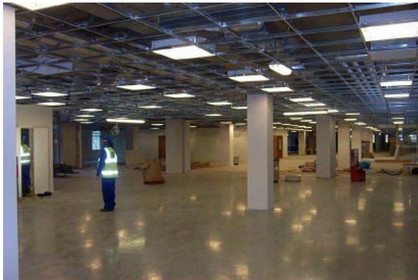
Figure 2: Example of internal fit out
