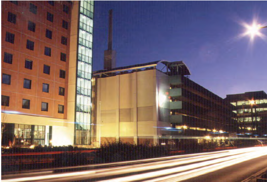
Woking Town Centre CHP District Energy Station - Thameswey Energy Ltd © Woking Borough Council
