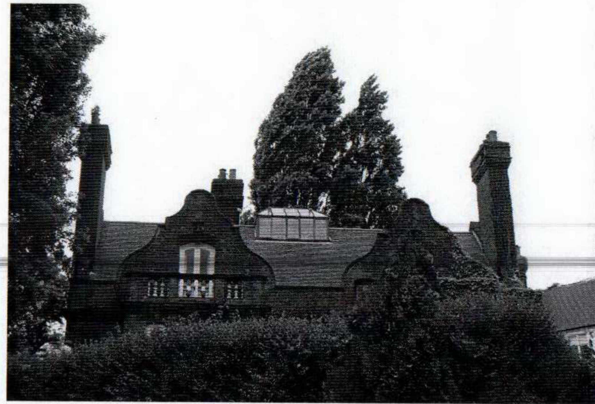
Existing lantern rooflight to no.4 Gainsborough Gardens
