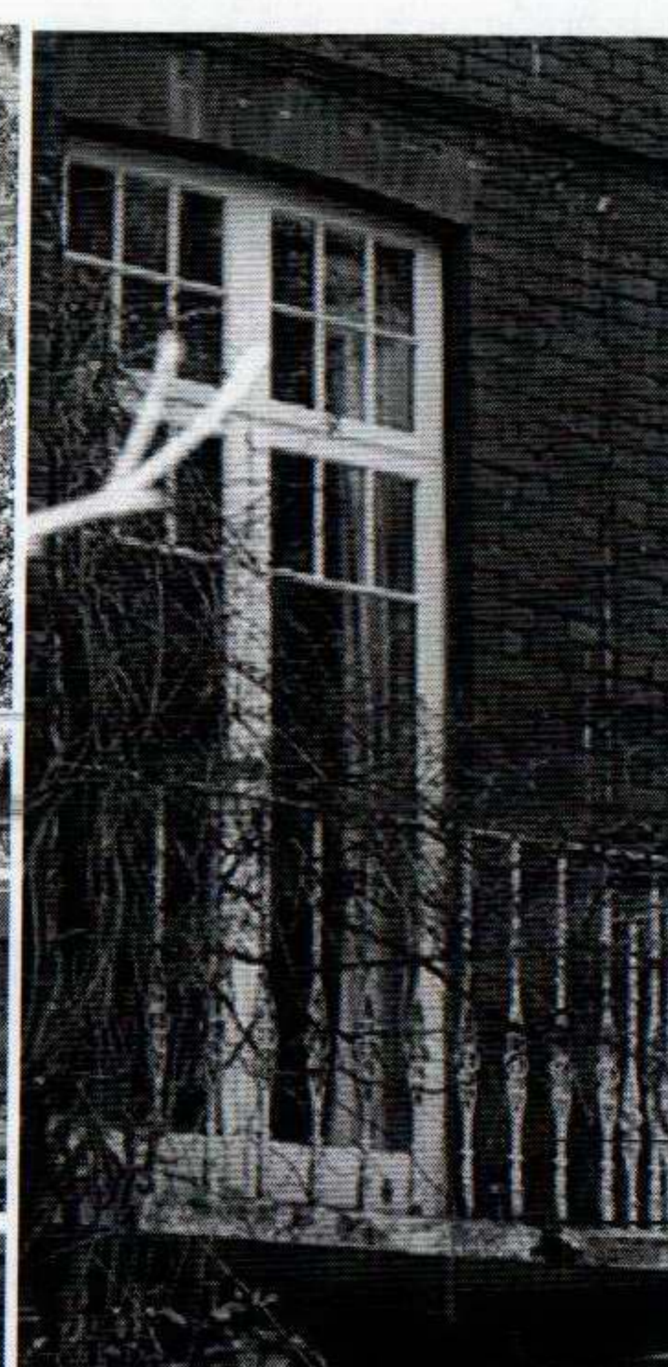
Balcony of no.9 Railings to be copied
