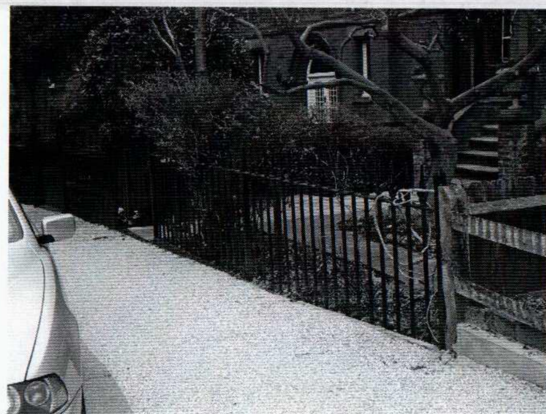
Adjacent neighbouring railings to be copied
