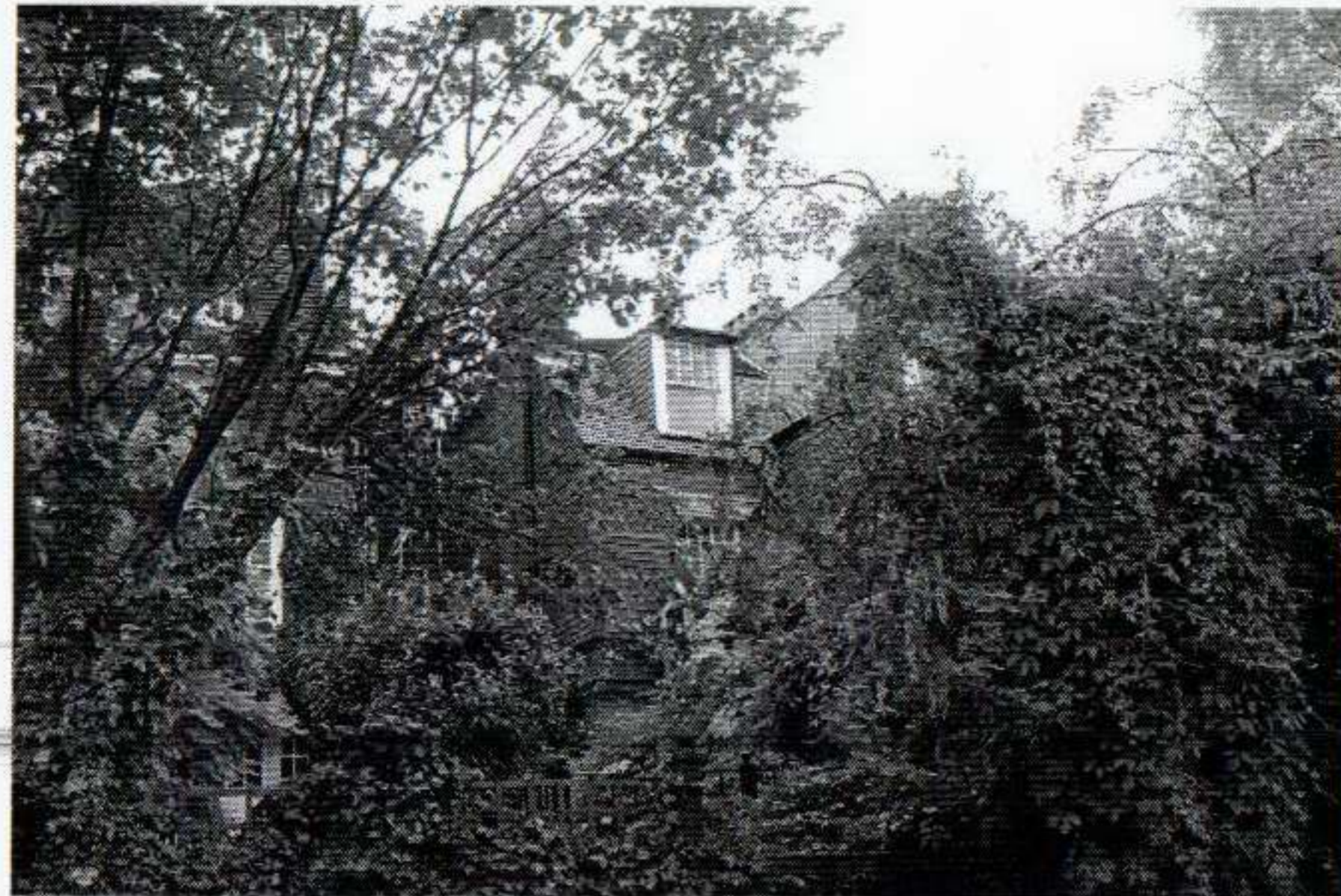
VIEW OF REAR OF GAINSBOROUGH GARDENS FROM CHRISTCHURCH HILL
