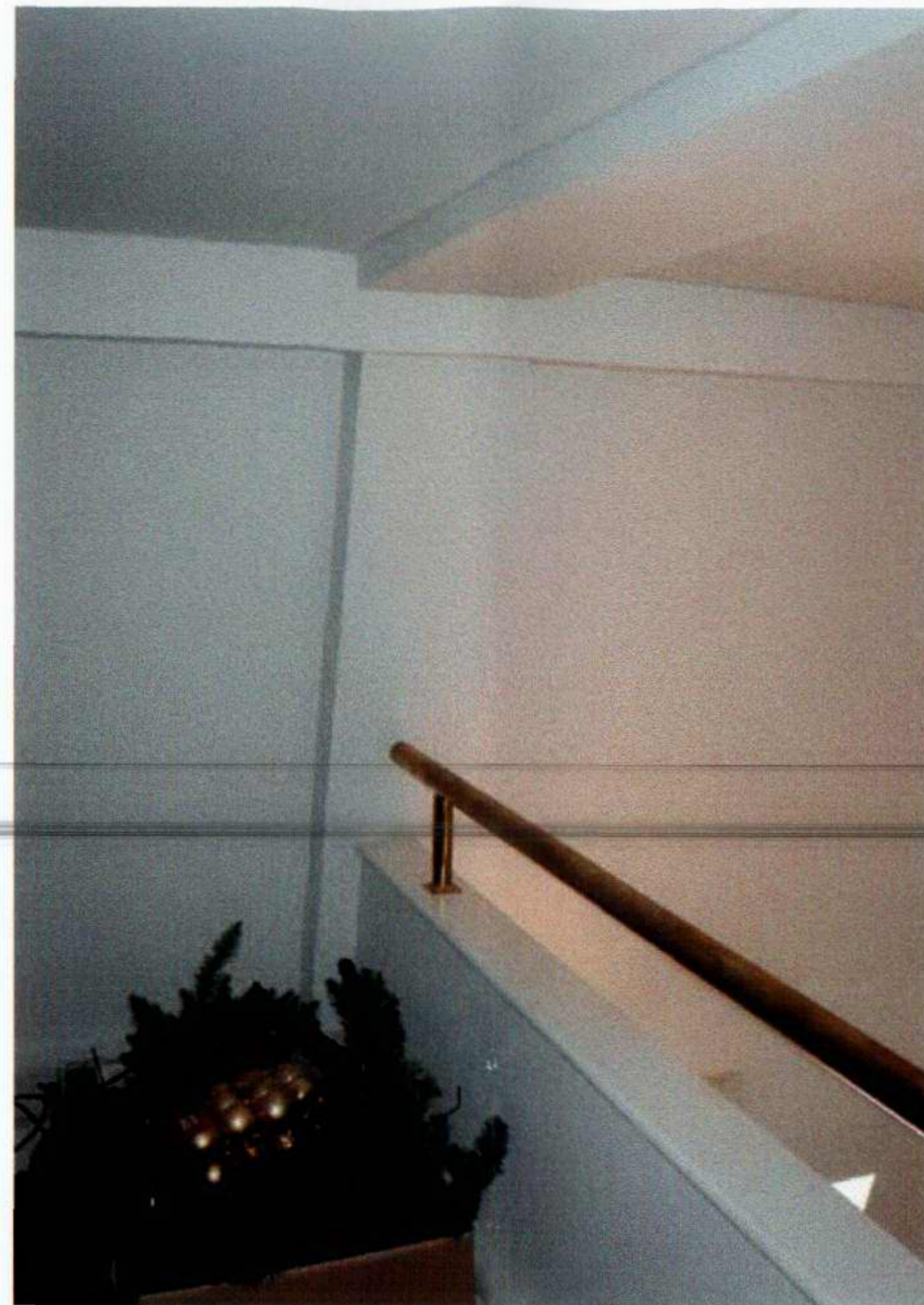
PH-1.02 View of existing balcony to 5th floor gallery space
