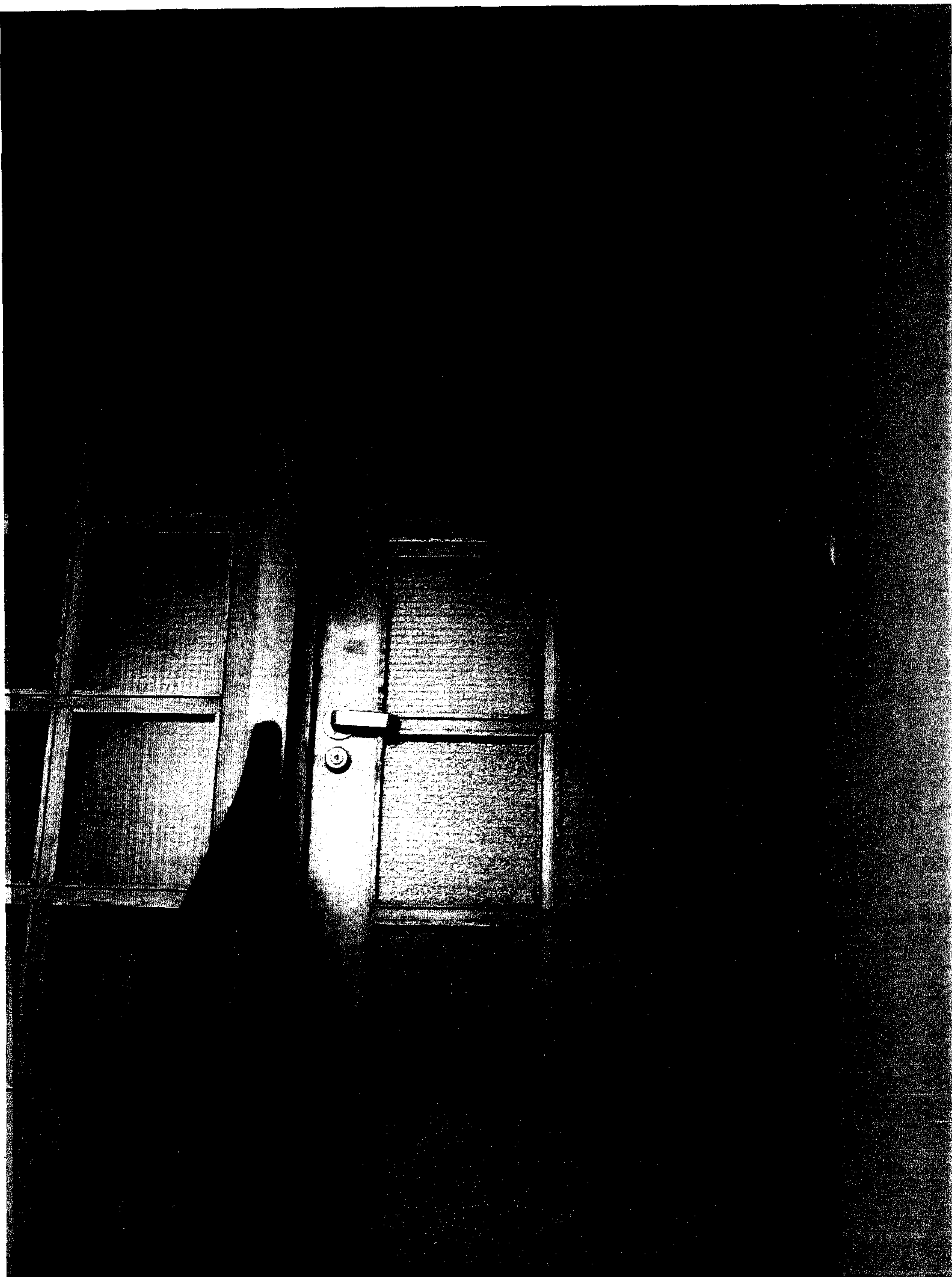
Entrance to flat 5 & 6 at 2nd floor (1930)
