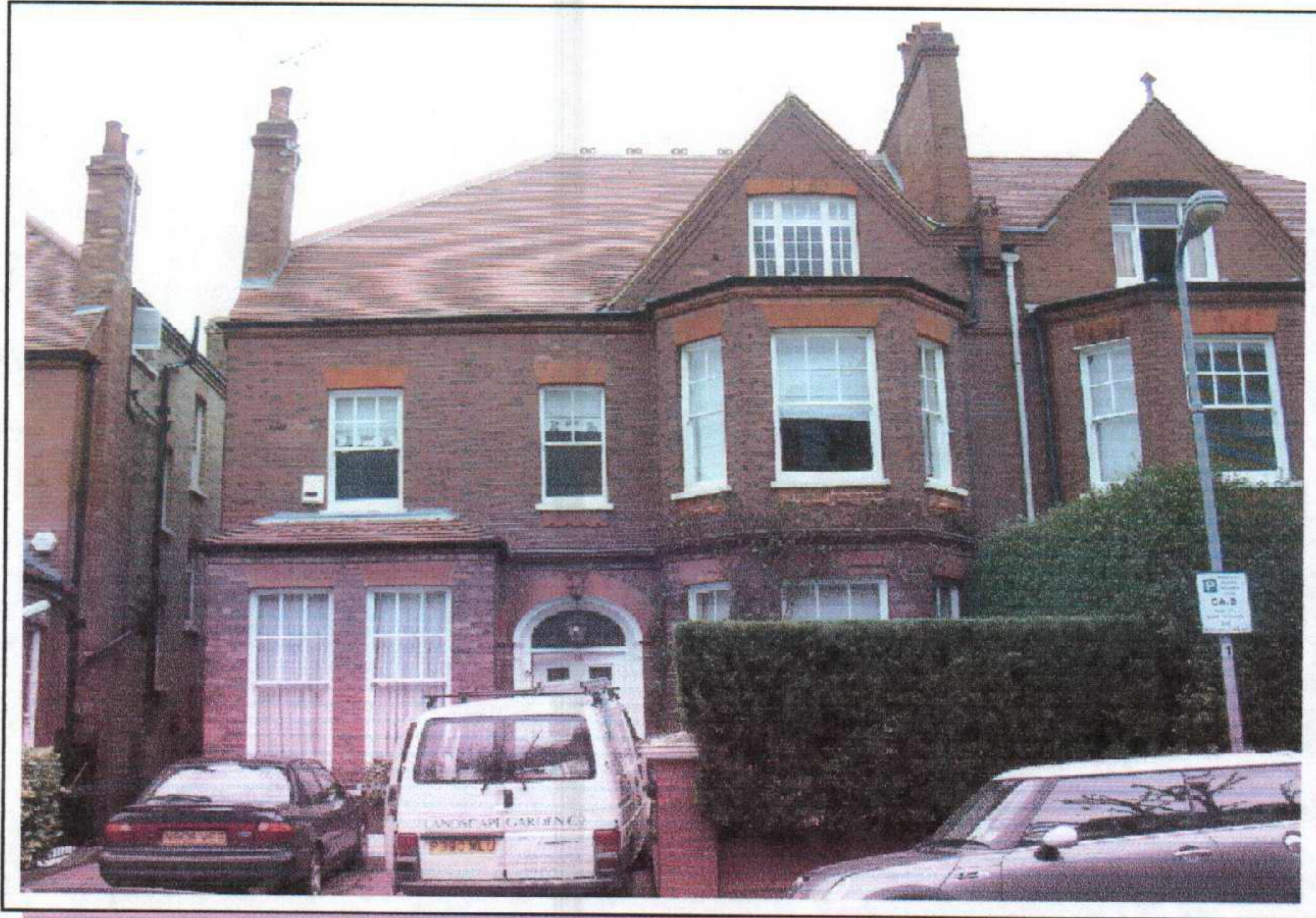
Photo 1: Existing front elevation
