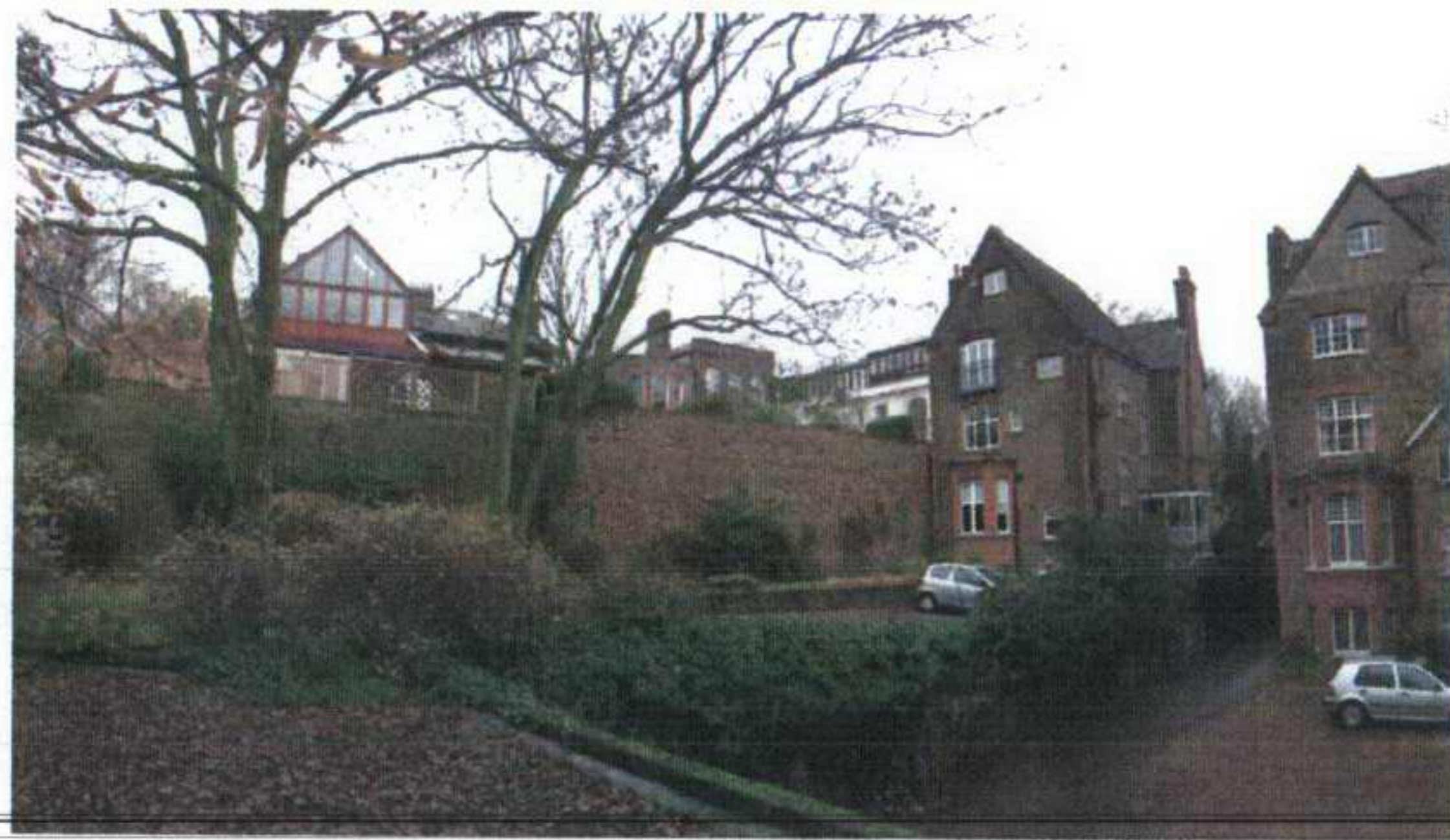
VIEW FROM TOP OF EXSITING GARAGE LOOKING NW
