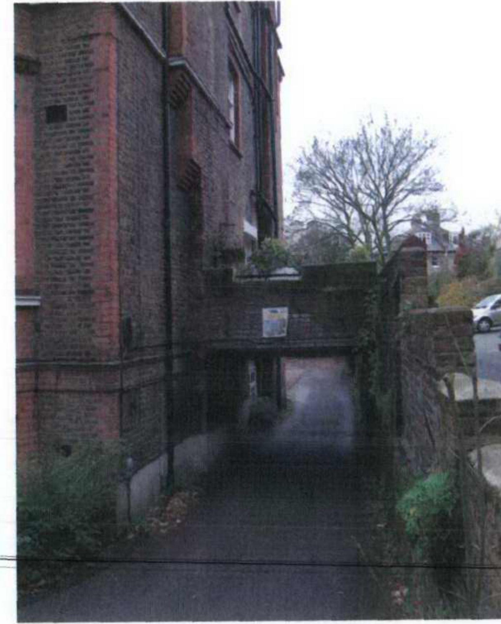
ACCESS TO THE REAR OF NO.19
