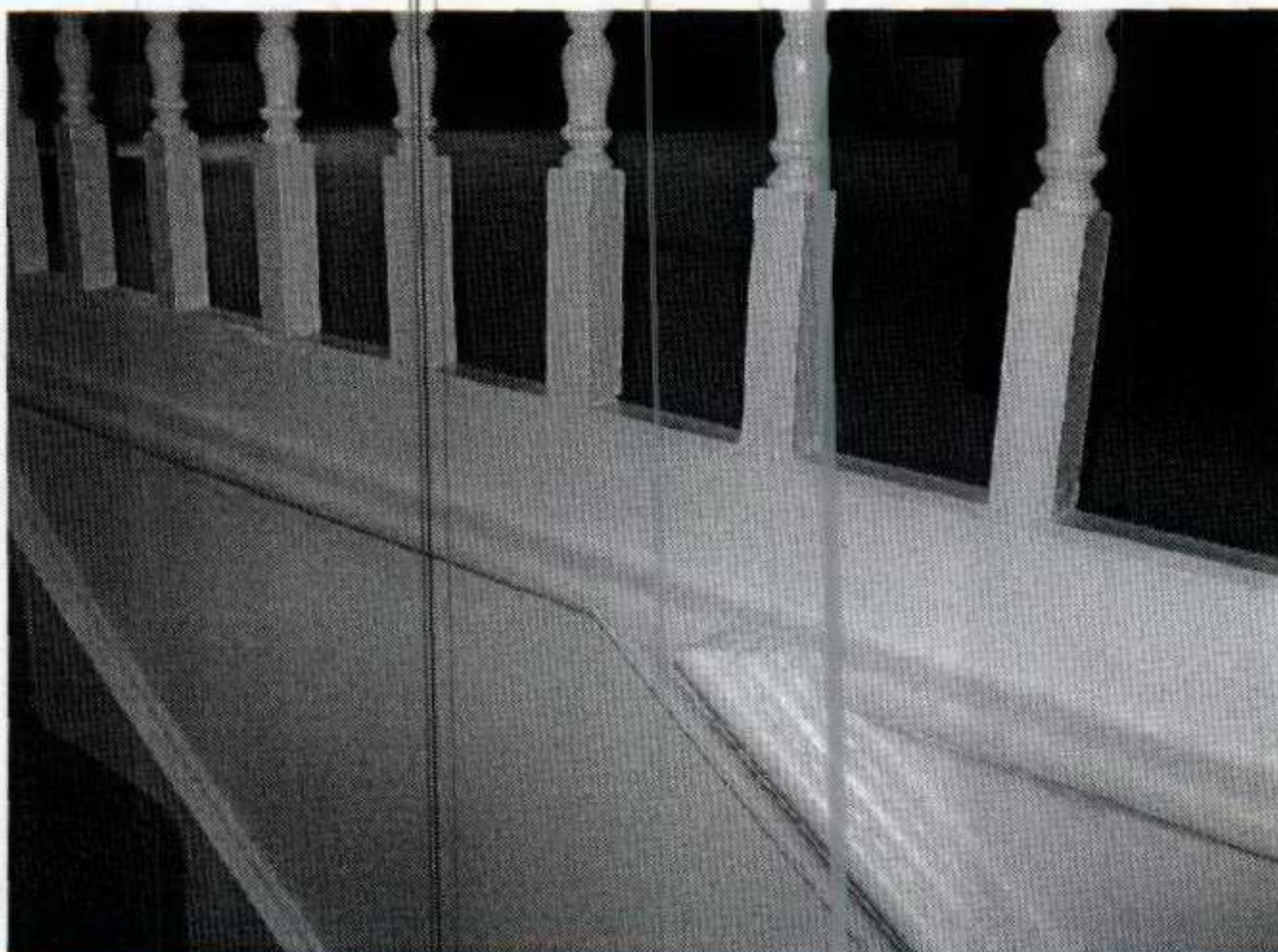
Photo 8 Balustrade base plate and string detail
