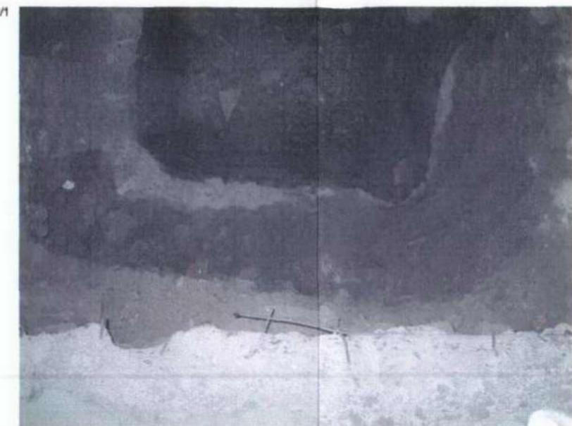
MATERIALS BELOW SLAB: BRICK WALL CONCRETE BASES RUBBLE INFILL
