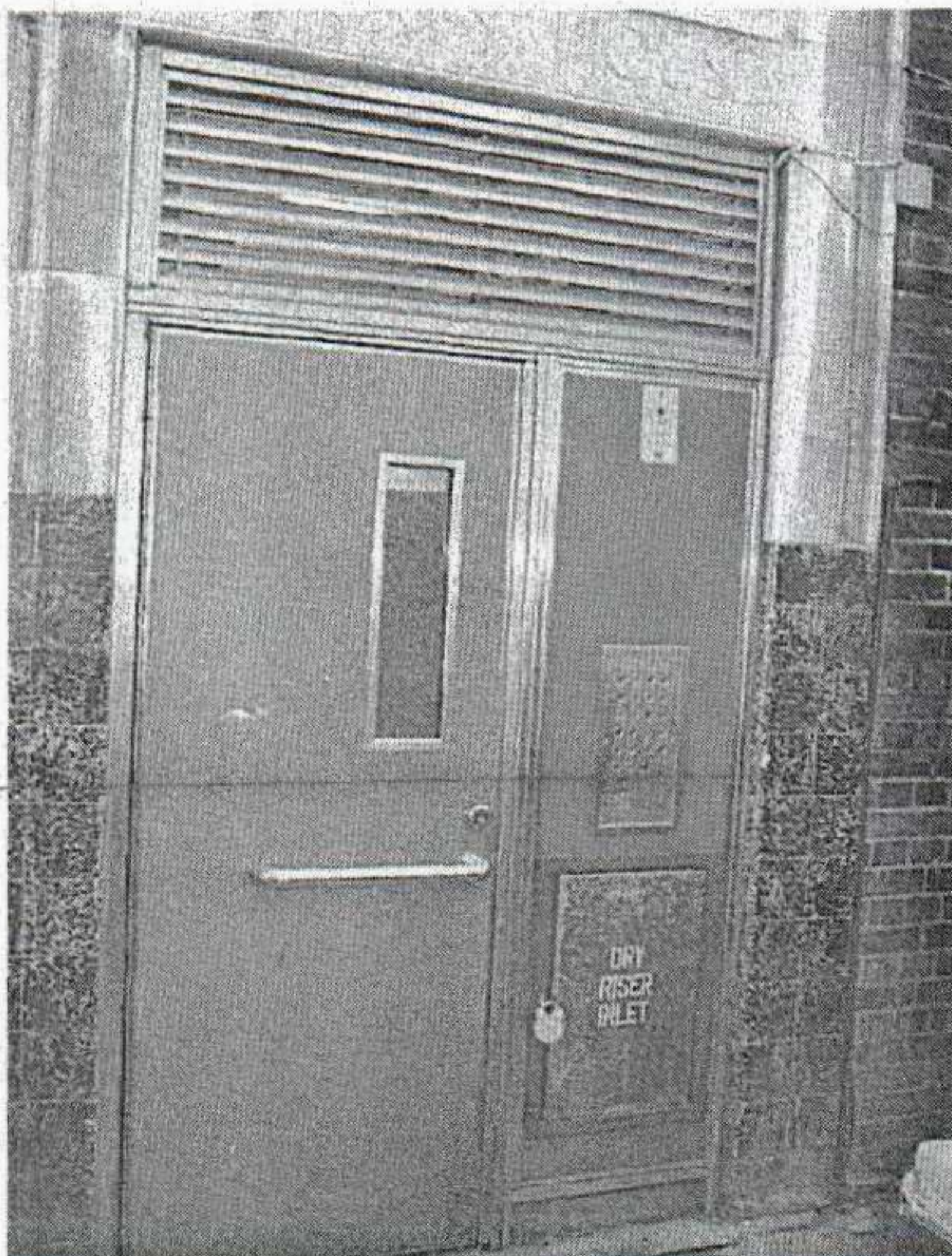
Existing front door
