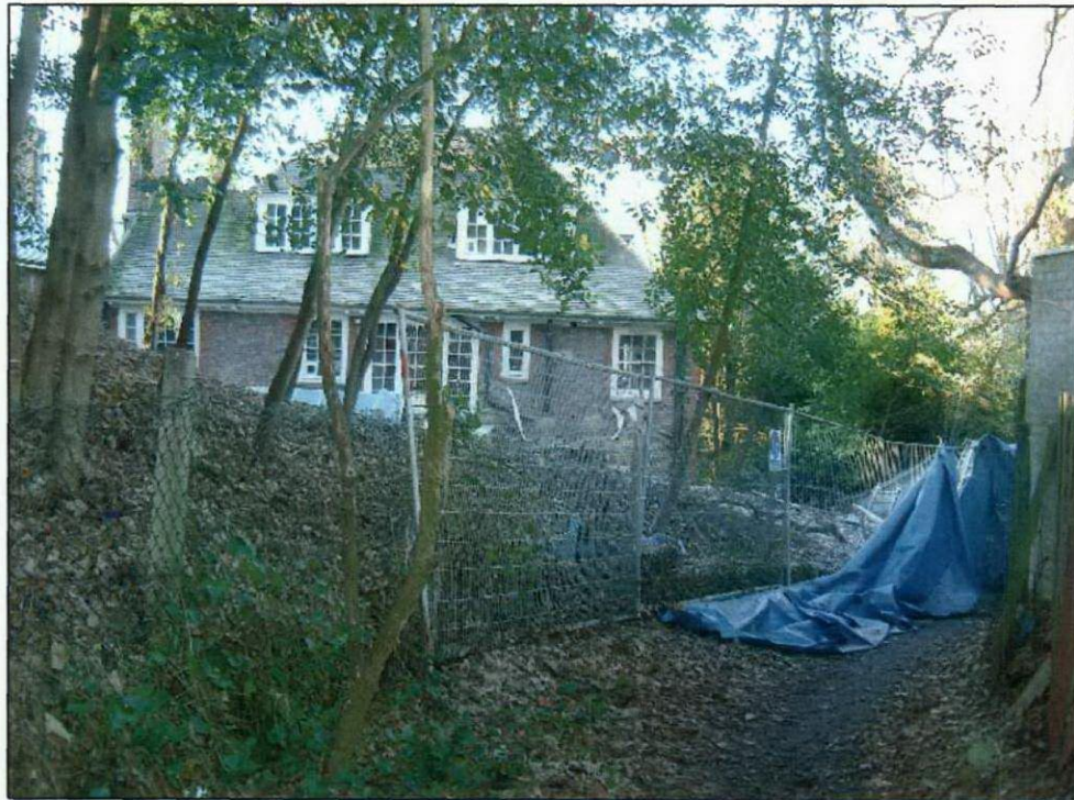
Rear Elevation viewed across high banked wooded copse from Oak Hill Way
