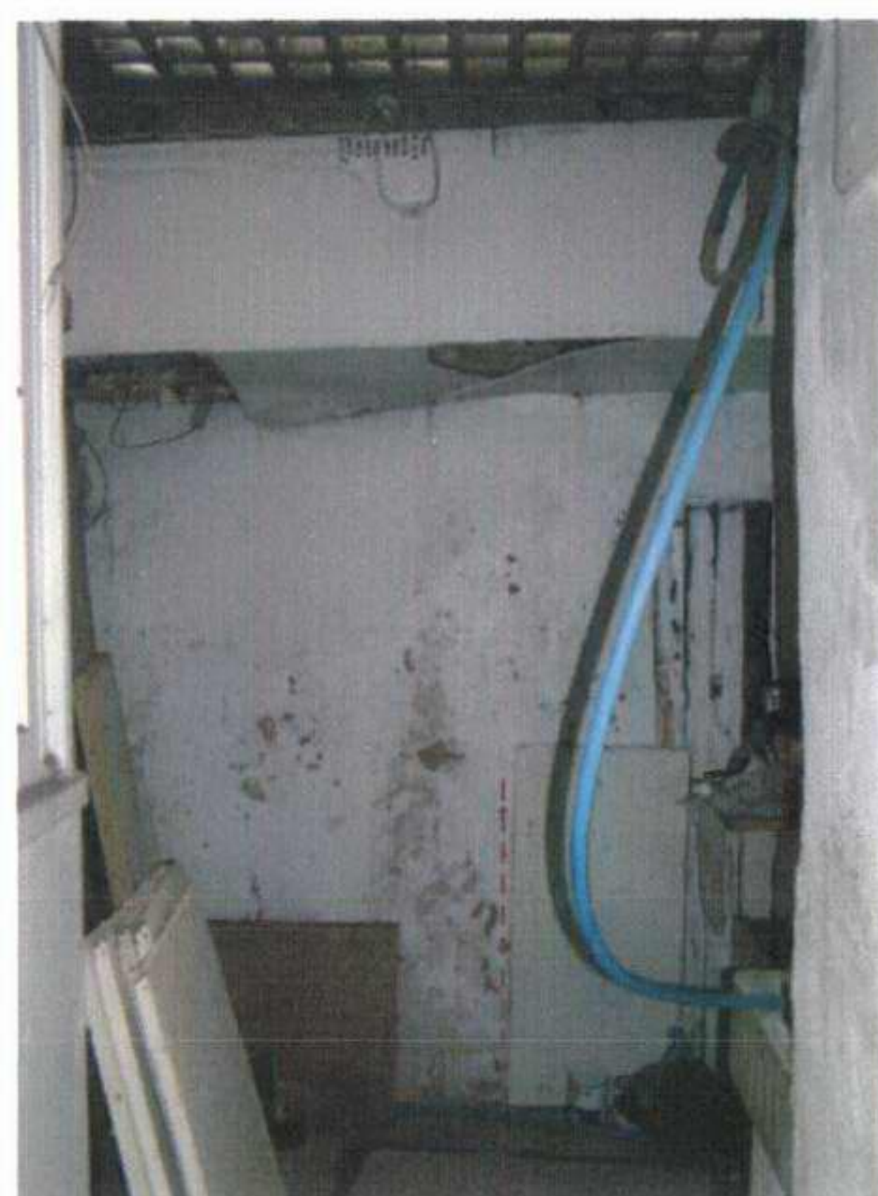
BASEMENT BEHIND W.C AREA
