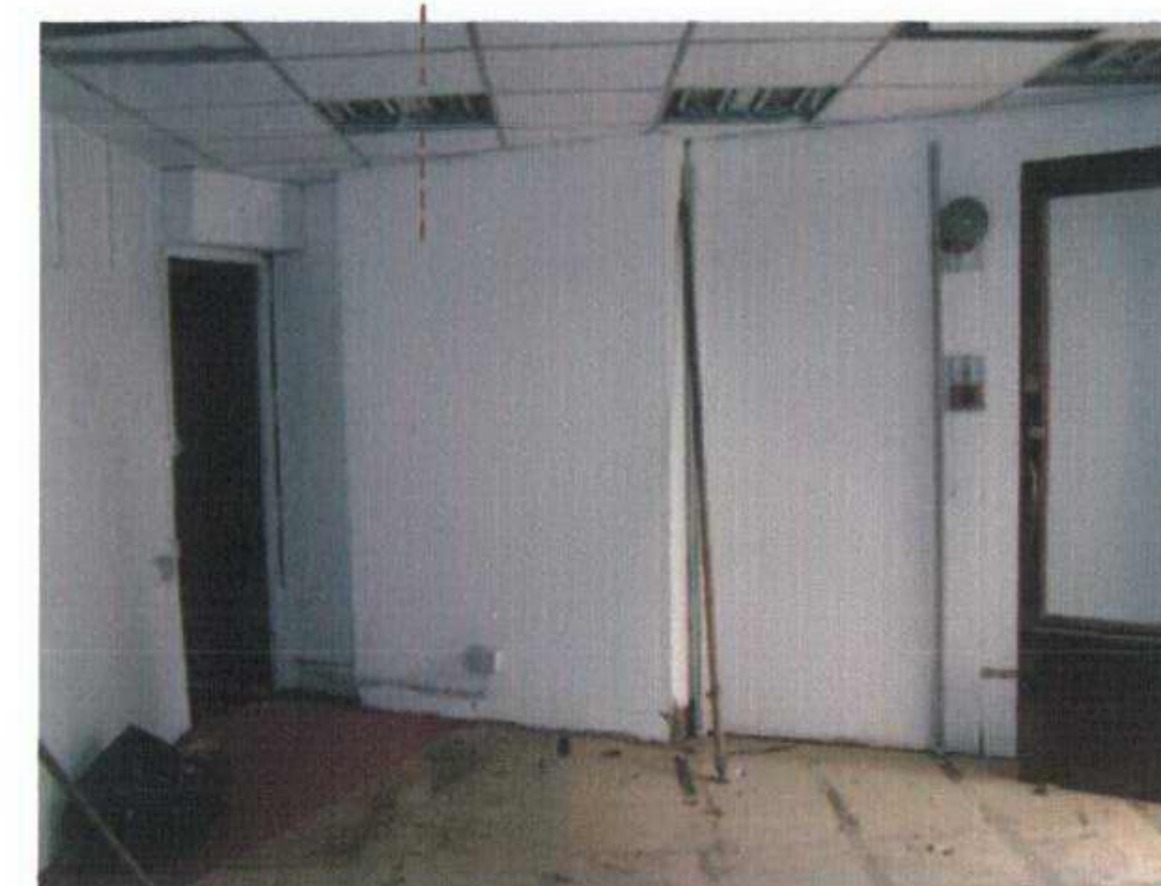
GROUND FLOOR NEXT TO ENTRANCE
