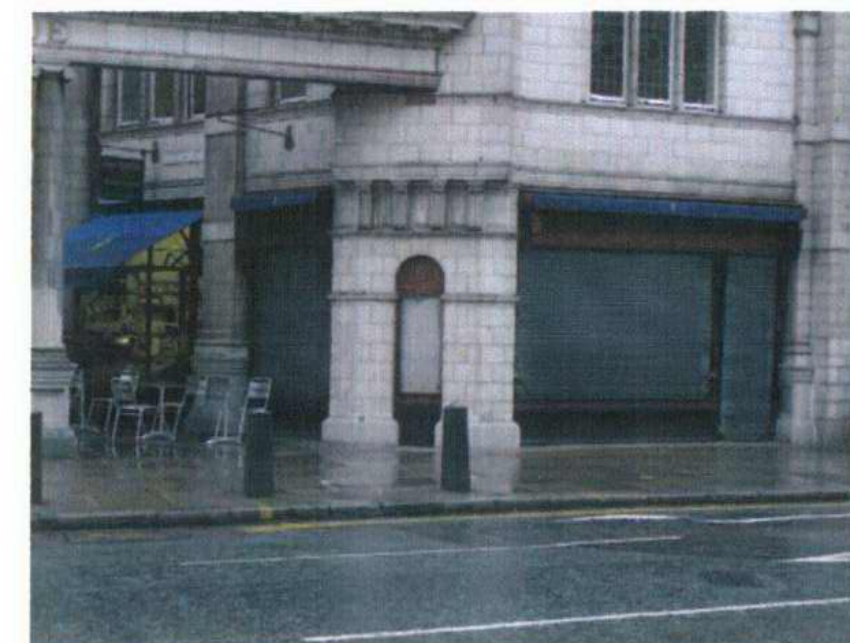
EXTERIOR VIEW LOOKING ONTO ENTRANCE OF 29 SICILIAN AVENUE
