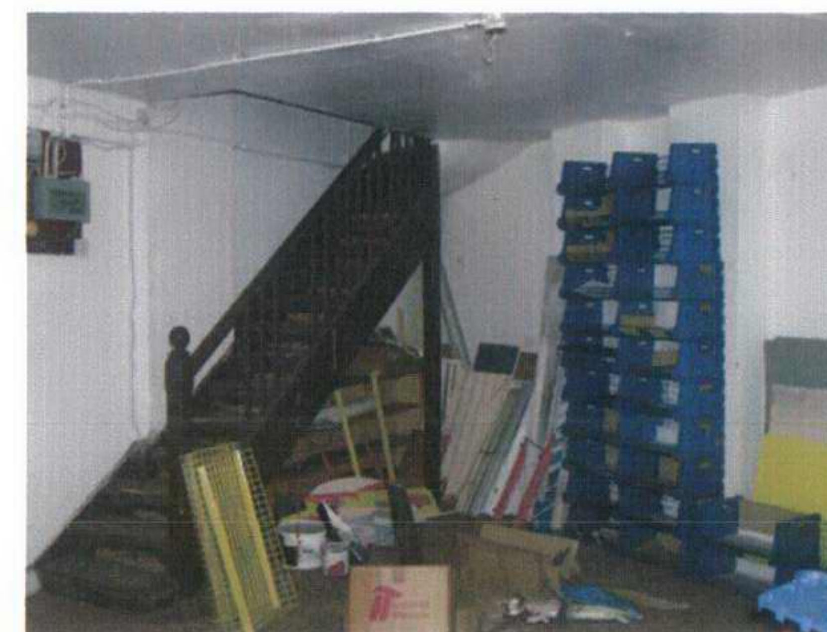
BASEMENT AND EXISTING STAIRCASE
