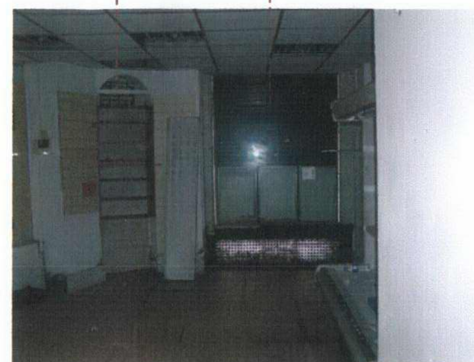
GROUND FLOOR EXISTING WINDOWS
