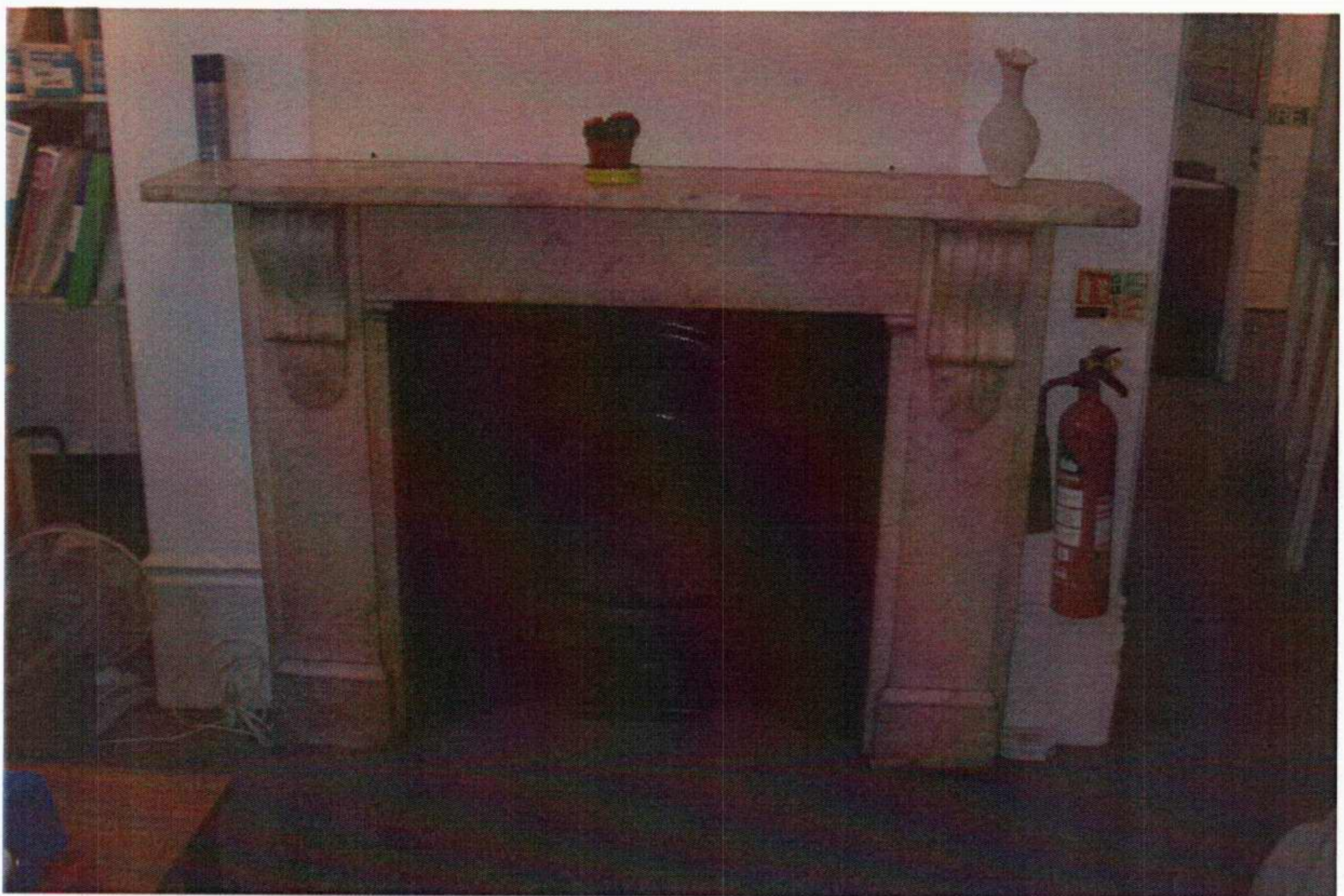
Fireplace to ground floor front room to be retained
