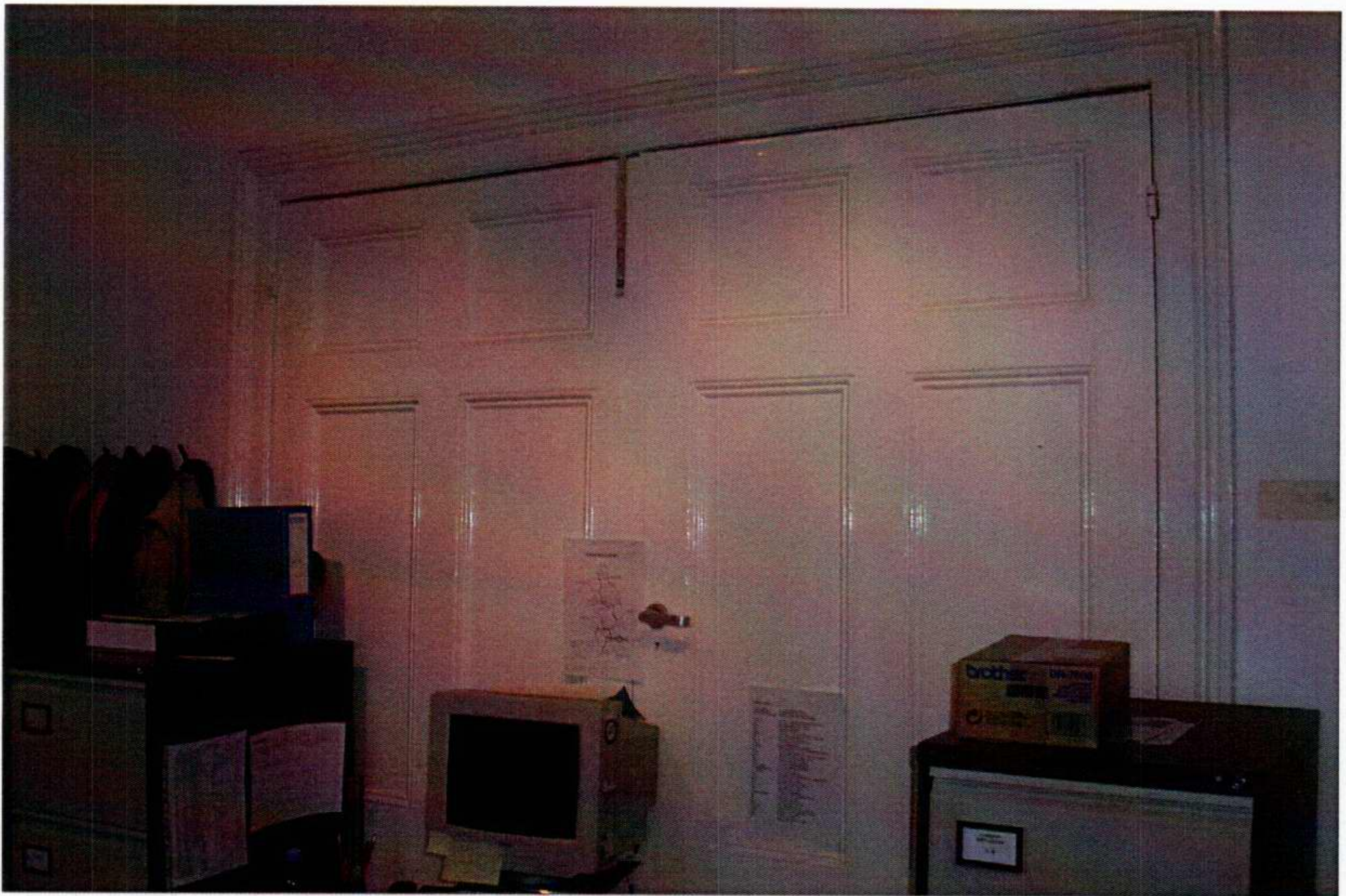
Original doors to ground floor spine wall to be retained
