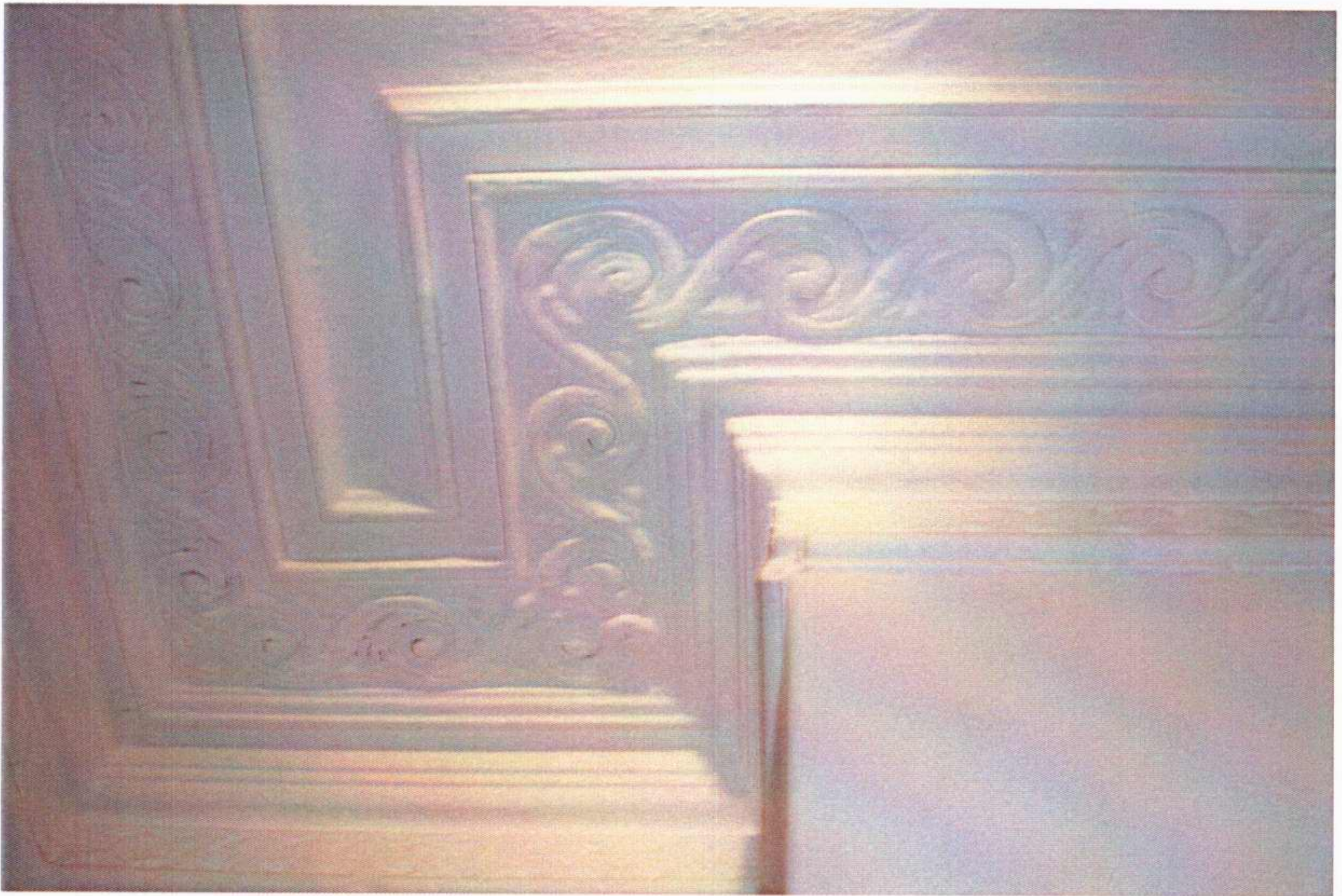
Ornate cornice to ground floor front room to be retained in full
