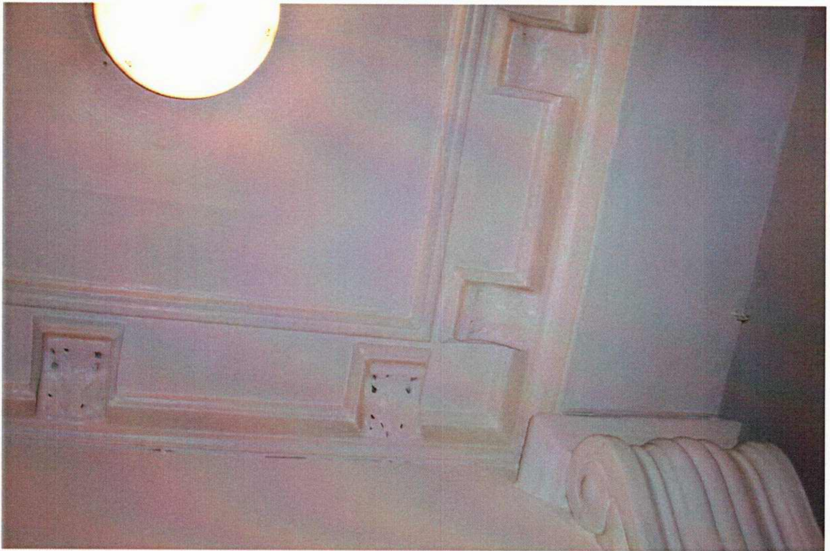
Ornate cornice to ground floor entrance to be retained in full
